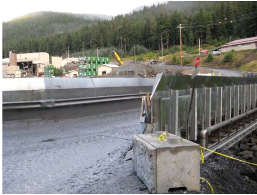
High splash walls on the bridge over Greens Creek outside the 920 portal.
