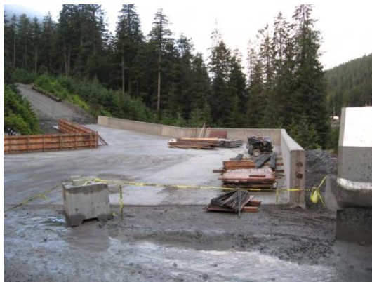
Concrete pads and walls to each side of the 920 mine entrance.
