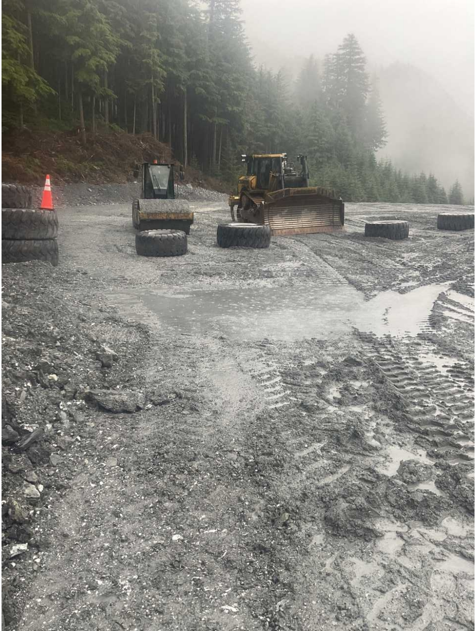
Photograph 2. Compacted Waste Rock at Site 23
