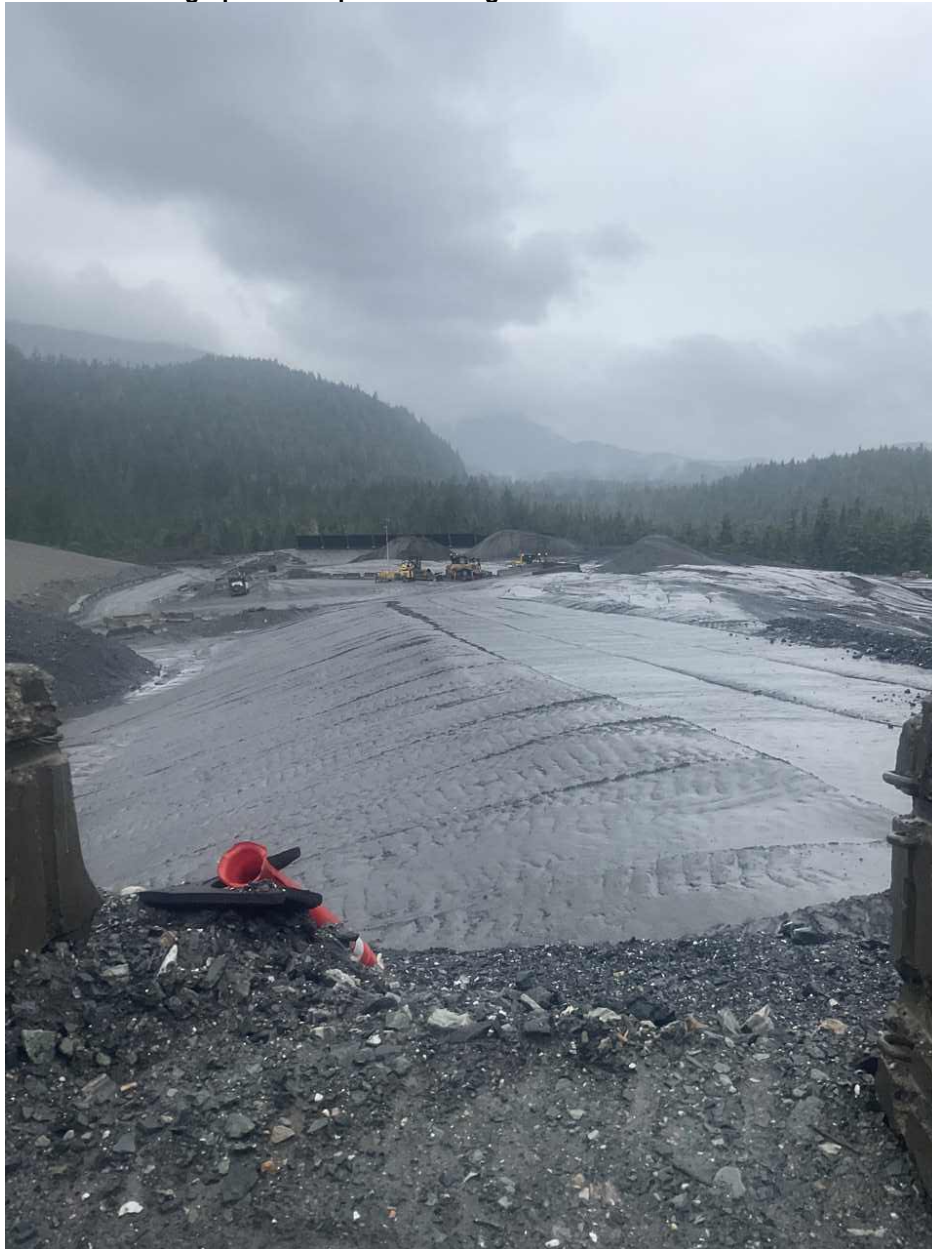
Photograph 1. Compacted Tailings and Waste Rock at the TDF
