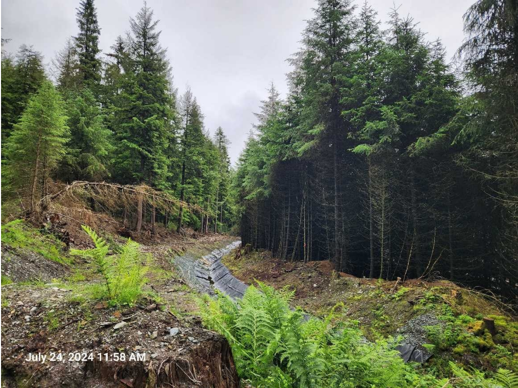
Photograph 9. New Drainage on Mill Backslope
