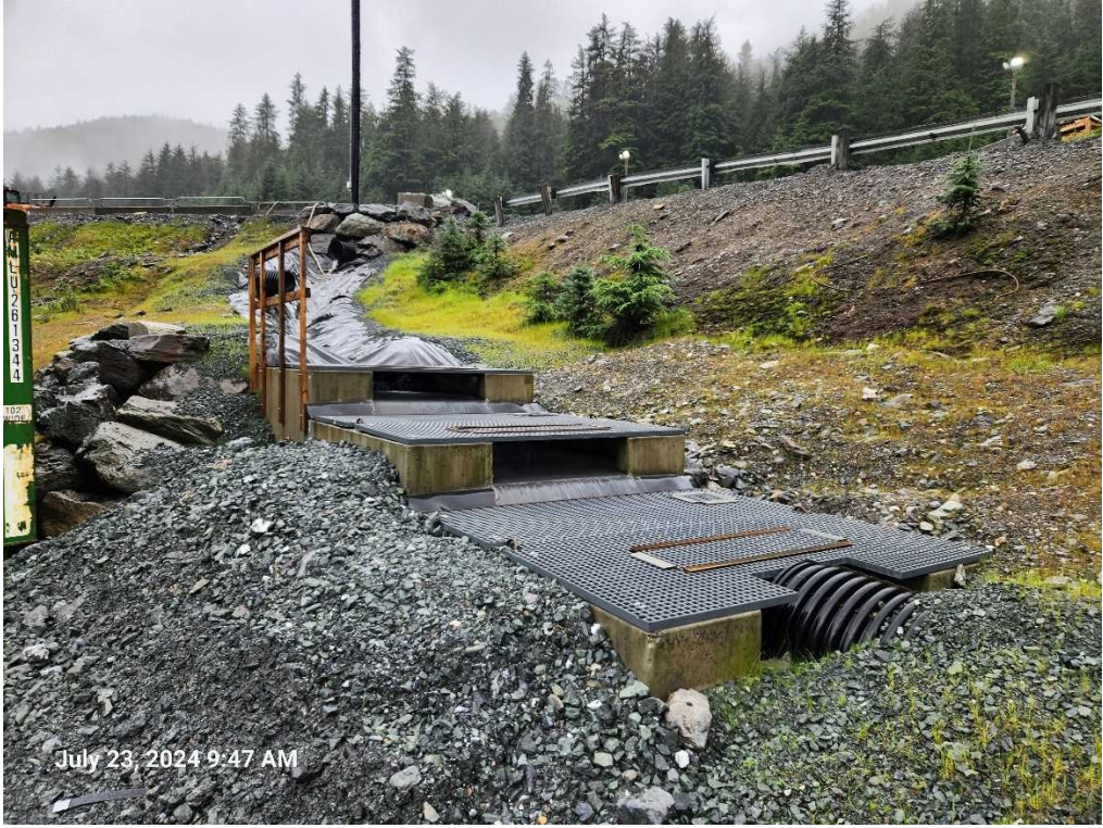
Photograph 10. New Sediment Capture Structure Near Ore Pad
