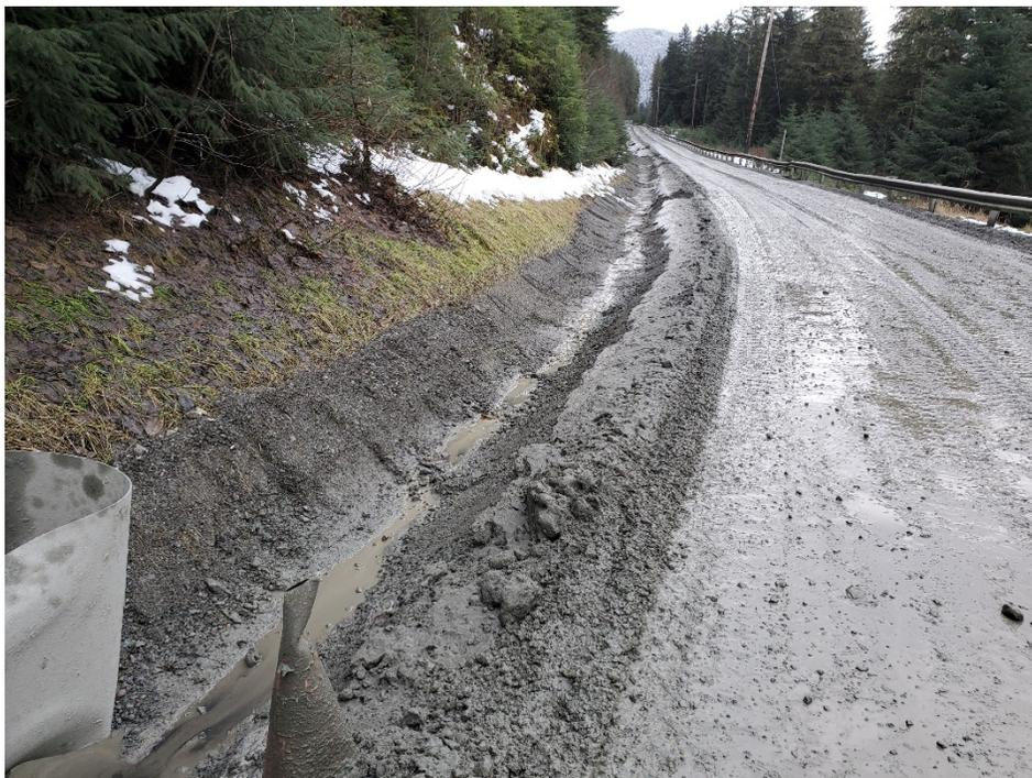
PHOTO 4. Repair of ditch above 3.4-mile bridge following 1 December storm.
