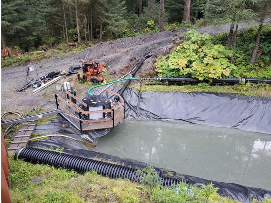
PHOTO 9. New discharge line from upper Pond C. Old piping remains in place as a backup.
