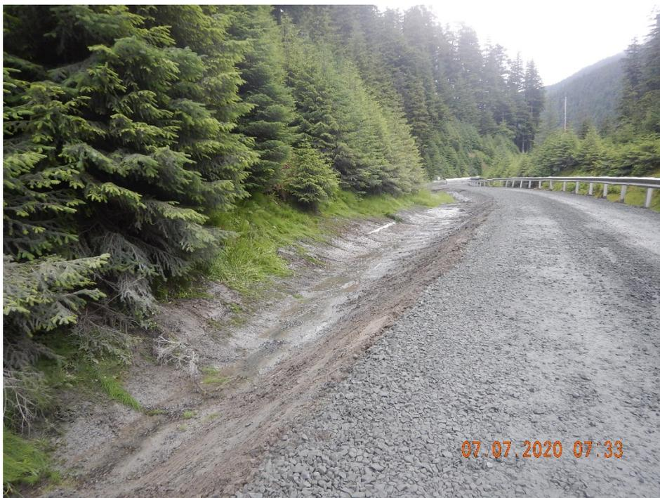
PHOTO 2. Road surface raised to establish a larger conveyance ditch for runoff.
