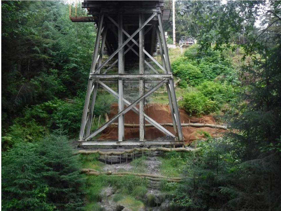
PHOTO 7. New straw wattles on south abutment of Zinc Creek bridge.
