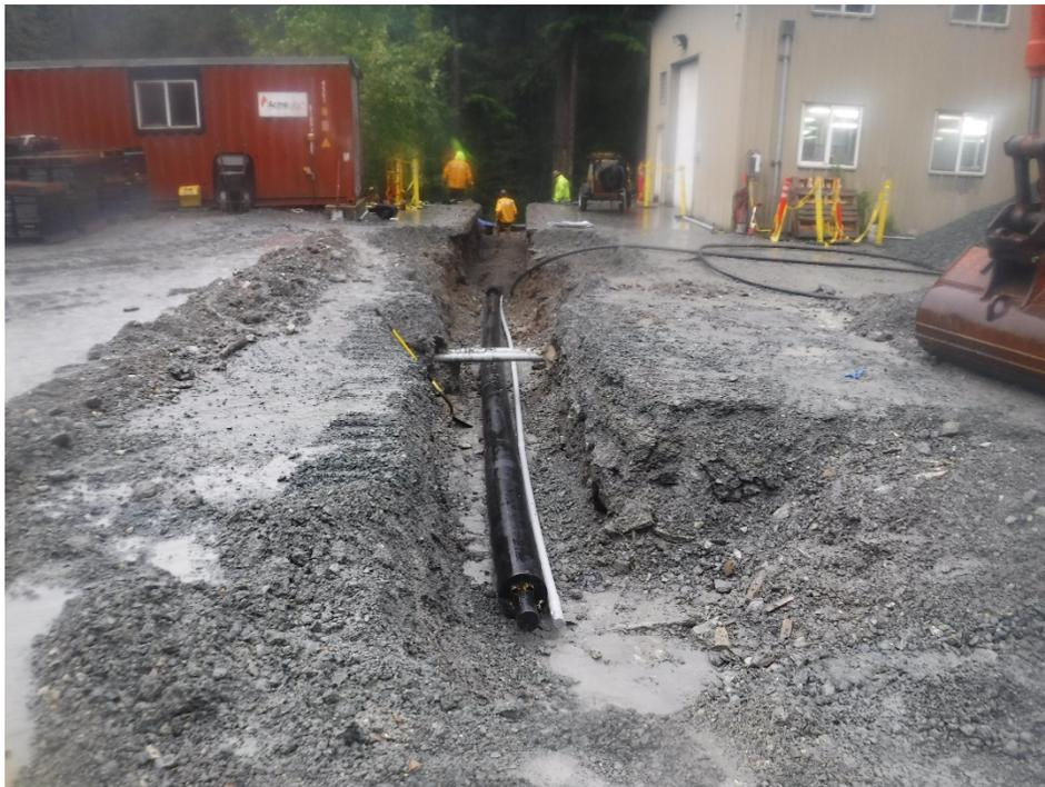
PHOTO 10. New discharge pipe being installed from upper Pond C.
