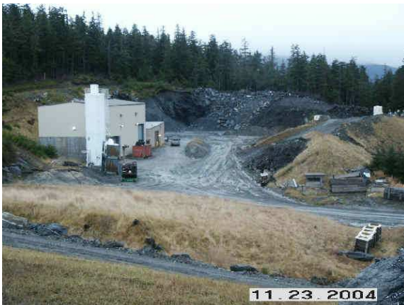
Waste Water Treatment Plant and Pit 5
