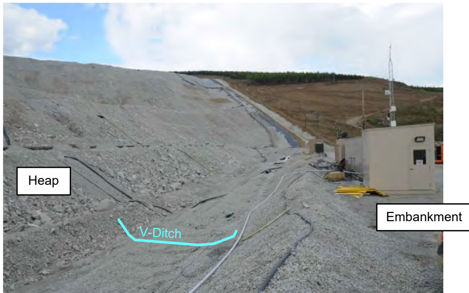
Figure 2-7 – V Ditch Looking North
