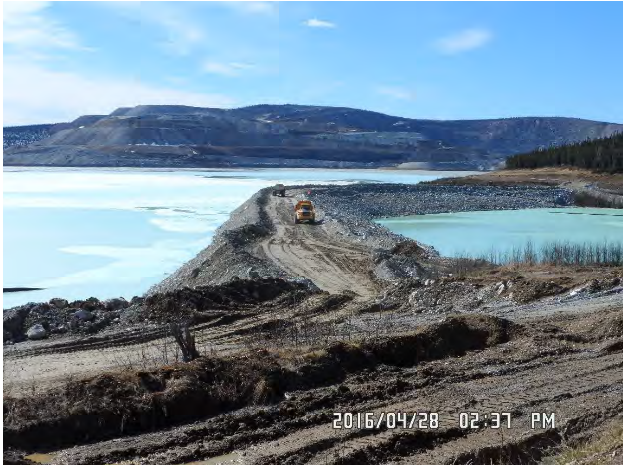
Figure 2-10 - Barge Pond Jetty
