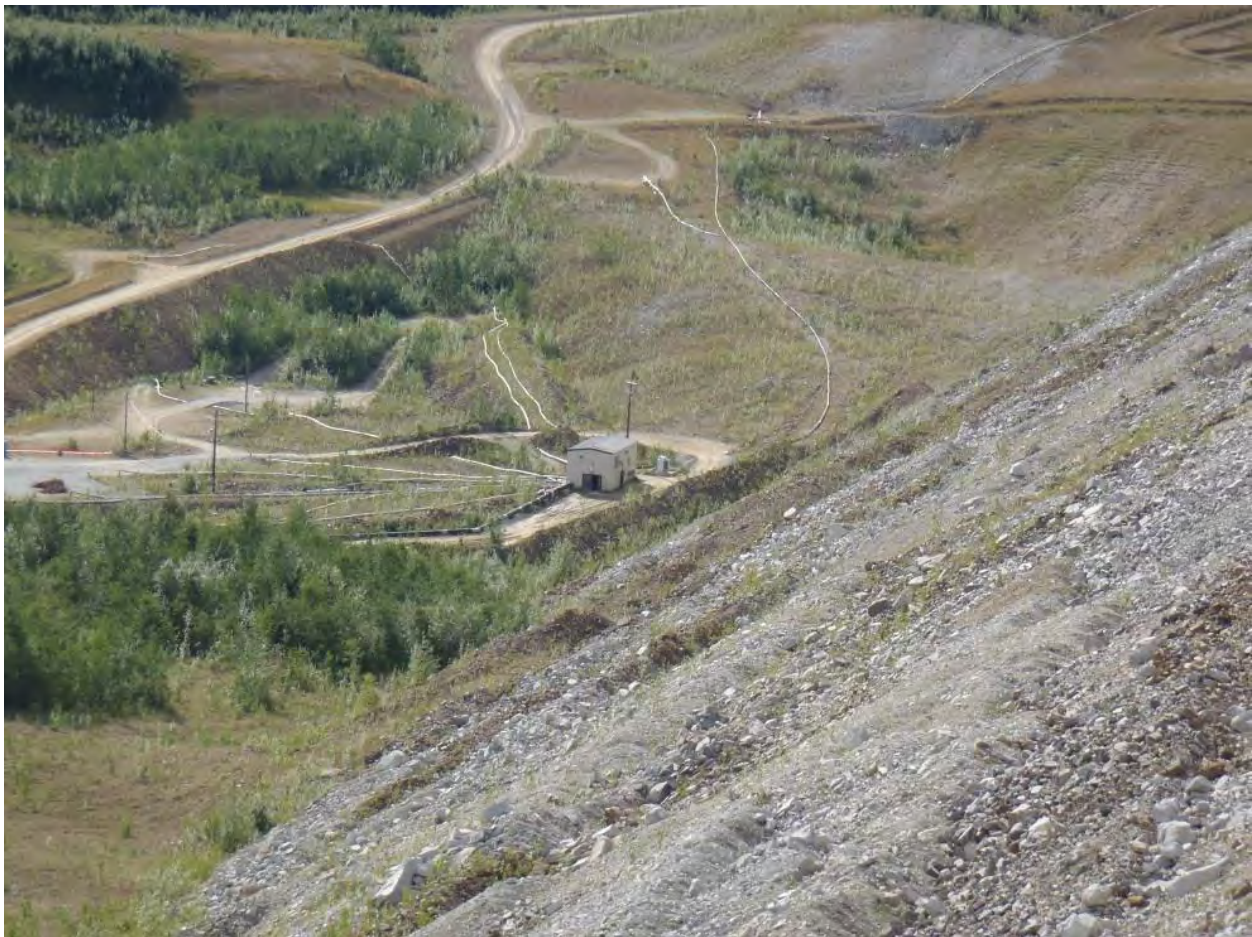
Figure 2-8 - Seepage Reclaim Building
