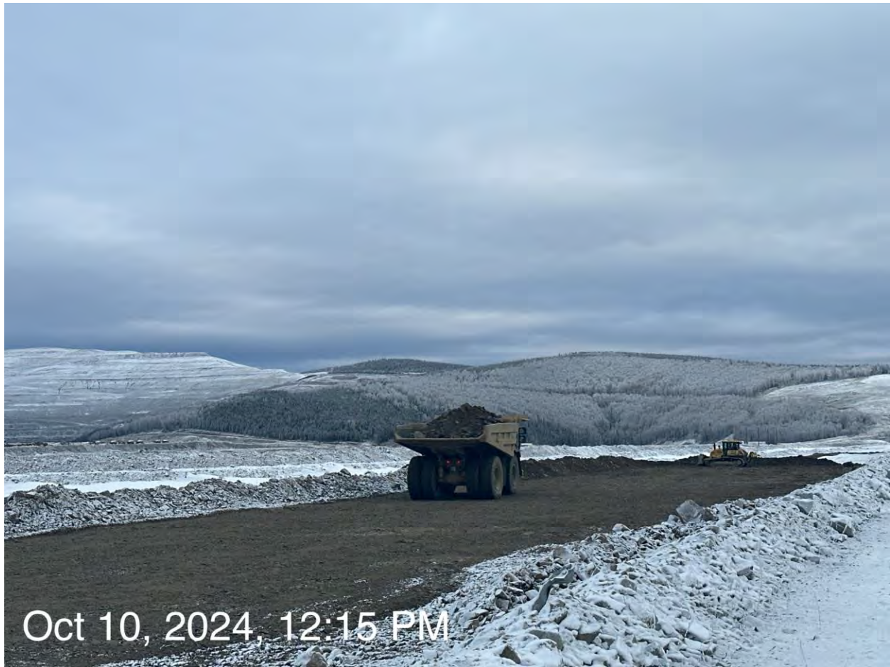
Figure 2-11 - Pearl Creek Causeway 2024 lift
