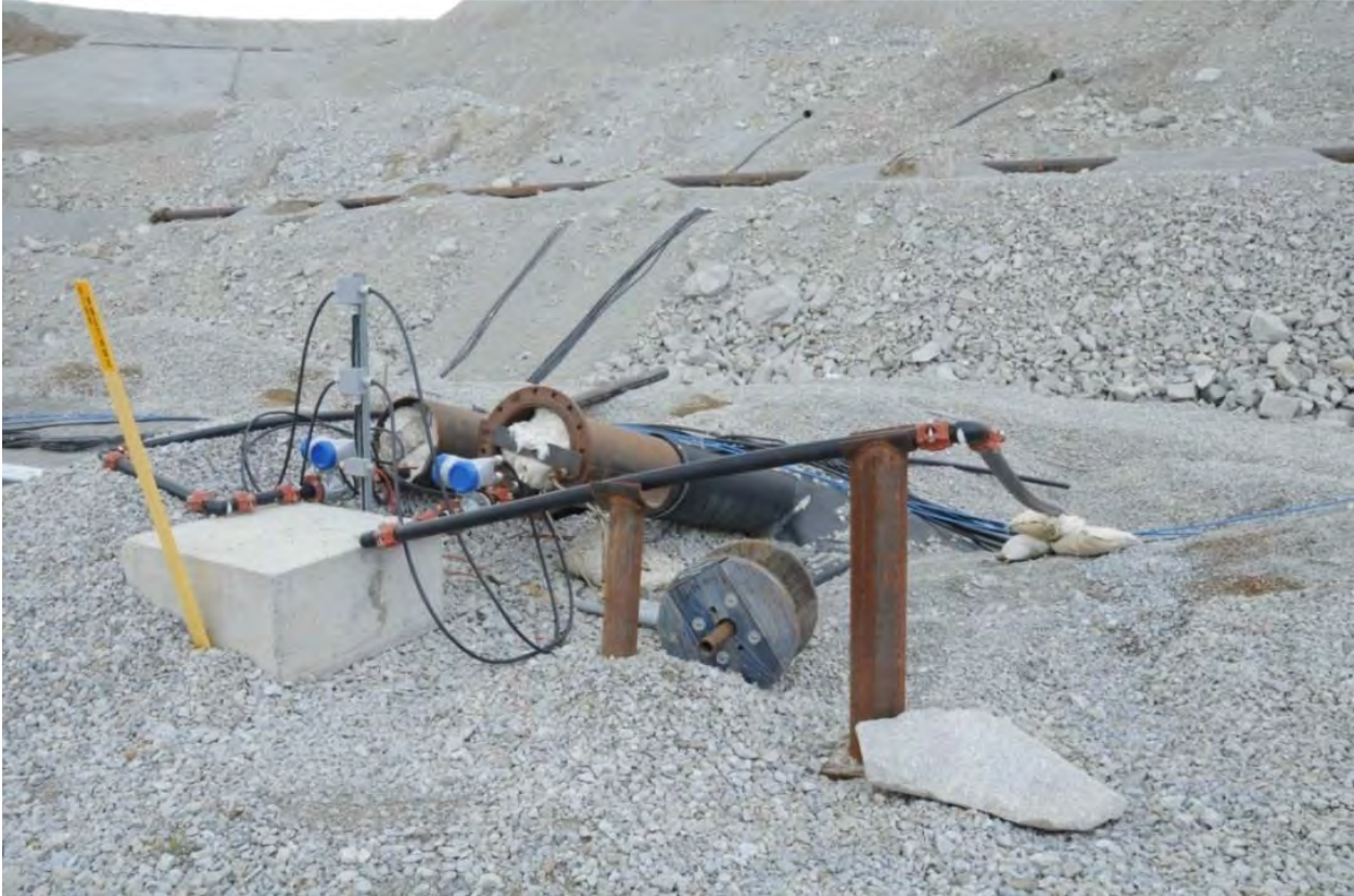
Figure 3-9 – LCRS Solution Collection Pipes
