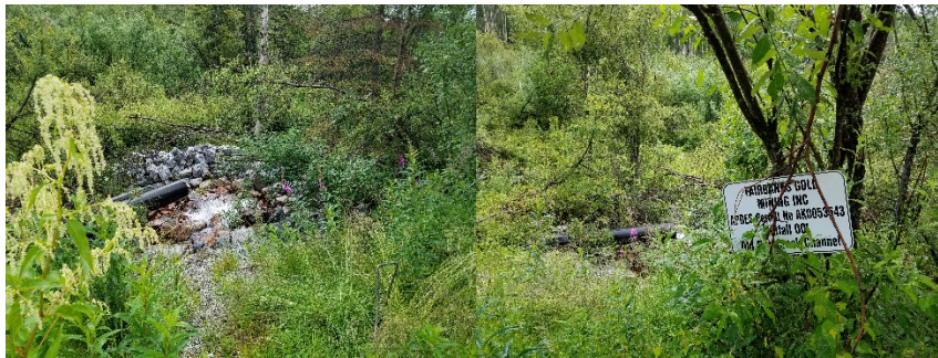
Outfall 001 – Reverse Osmosis Water Treatment Plant (RO1)
