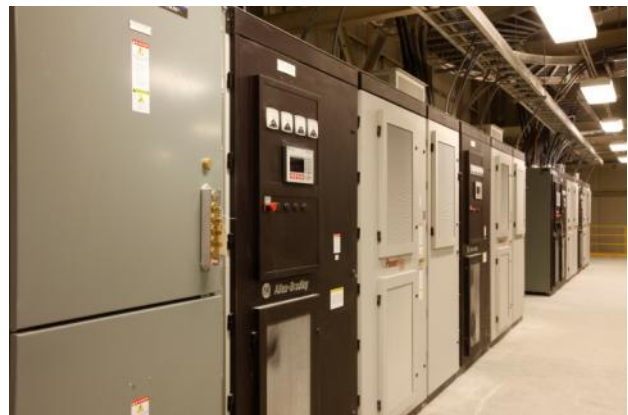
The SAG mill drive was upgraded in 2009.
