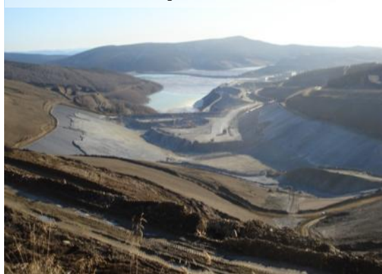
Walter Creek heap leach construction
