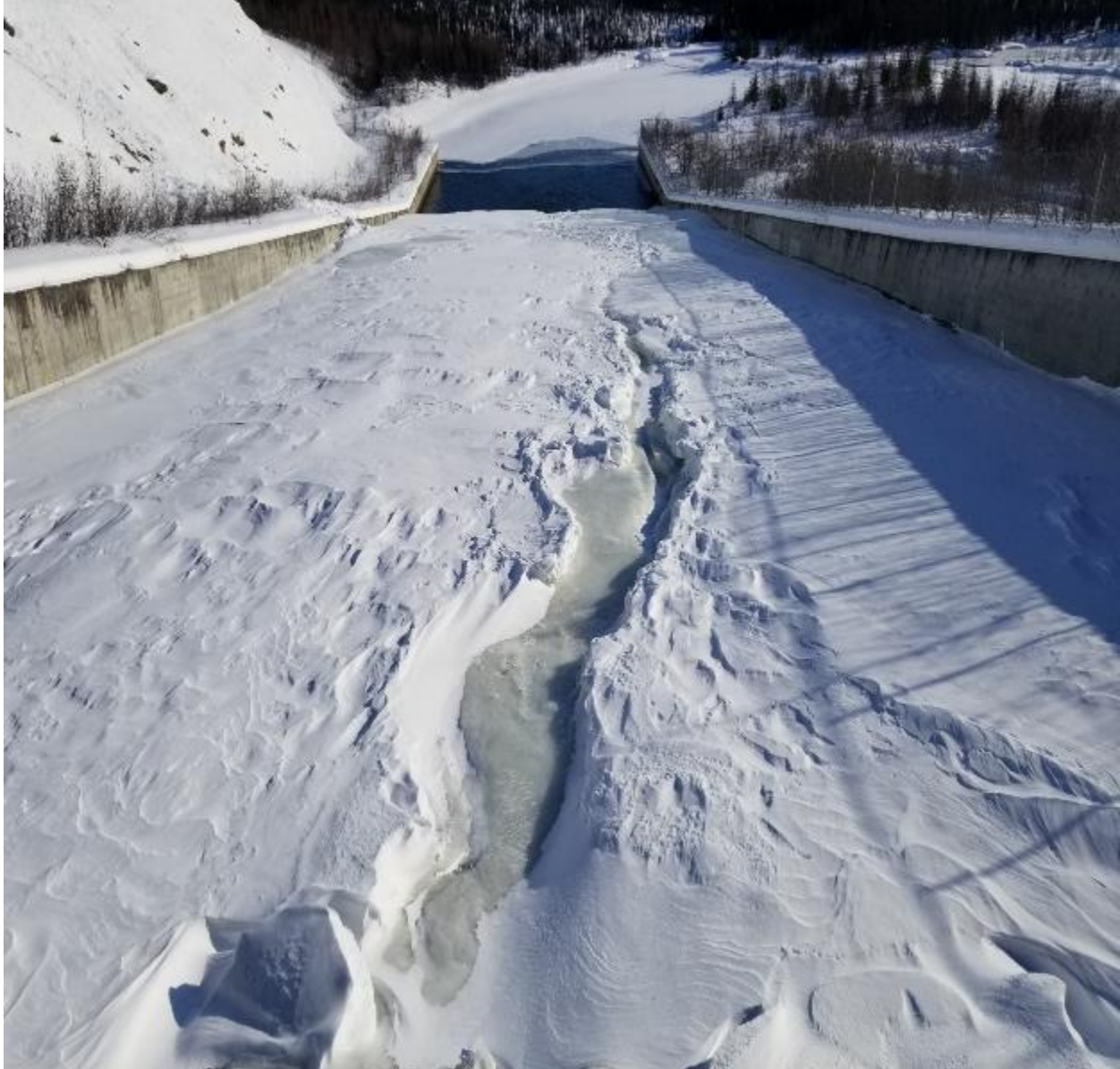
Figure 4. Spillway at outlet of Water Supply Reservoir on April 10, 2020.
