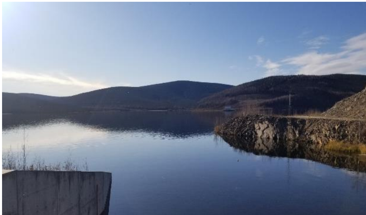
Figure 2. Fort Knox Water Supply Reservoir (WSR) October 2020.
