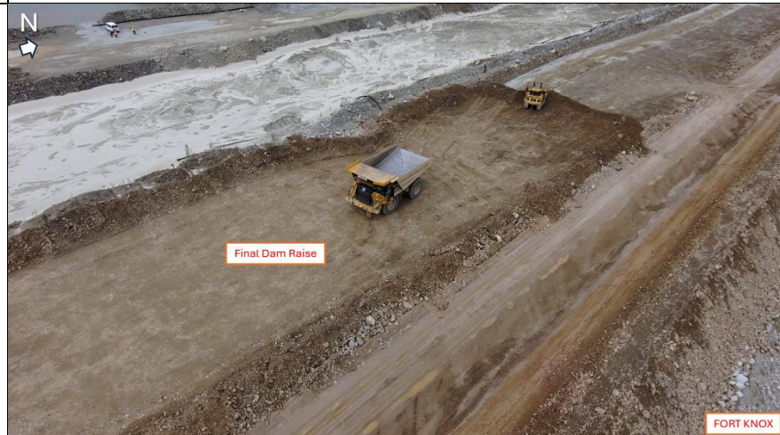
Photo 20: TSF Dam and view of final dam raise active construction.
