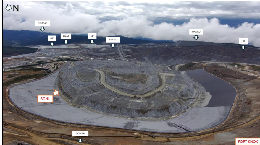
Photo 10: Barnes Creek HL and lower levels of the WRD with distant views of the south Fort Knox pit wall, Yellow Pup and Fish Creek WRDs, North and South ponds separated by the Pearl Creek Causeway, and TSF Dam and distant view of the Gil Road.
