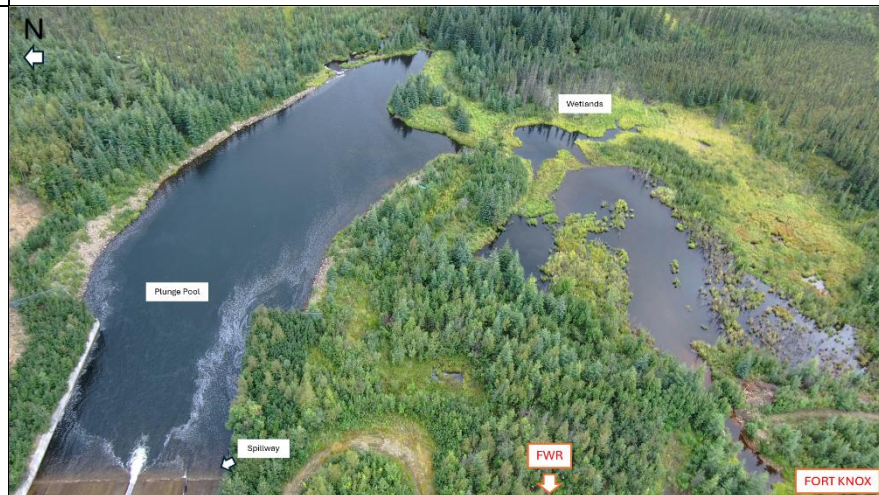
Photo 34: FWR spillway, plunge pool, and wetlands.
