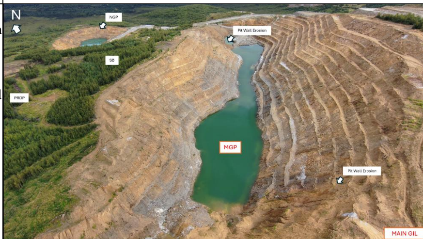
Photo 24: Main Gil Pit exhibiting pit wall erosion and groundwater inflill. Note the location of the Snack Bar, Partially Reclaimed Drill Pads, and North Gil Pit
