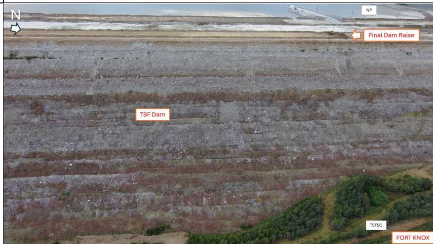
Photo 22: Western view of the TSF Dam including final dam raise.
