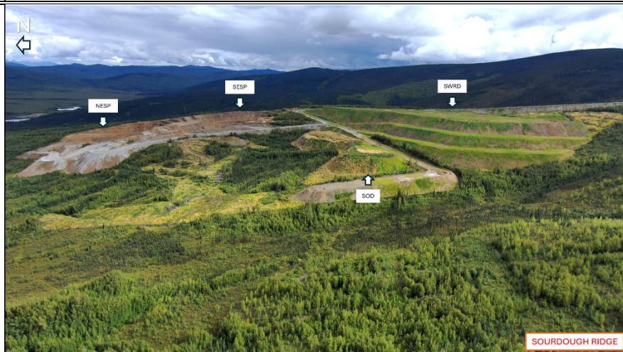
Photo 30: View of Sourdough Ridge from Main Gil including Northeast Sourdough Pit (NESP) and Southeast Sourdough Pit (SESP), Sourdough Waste Rock Dump (SWRD), and Sourdough Organic Dump (SOD).
