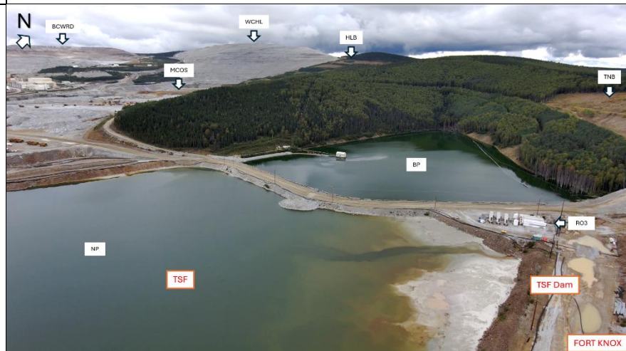
Photo 18: Barge Pond and RO3 Water Treatment Plant including views of the dam crest, North Pond, Tailings North and HL borrows, Manh Choh Ore Stockpile, Walter Creek HL, and Barnes Creek WRD.
