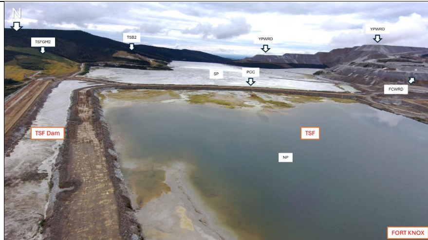
Photo 17: Tailings Storage Facility with views of Pearl Creek Causeway, North and South ponds, dam crest, Fish Creek WRD, upper and lower portions of the Yellow Pup WRD, Tailings South Borrow 2, and TSFGM2.
