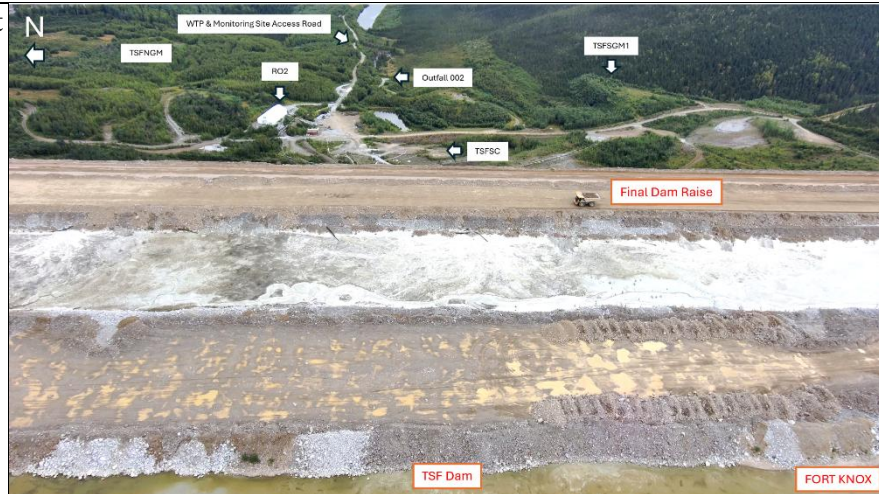
Photo 19: TSF Dam crest and final dam raise including views of RO2 Water Treatment Plant, Outfall 002, and GM stockpiles.
