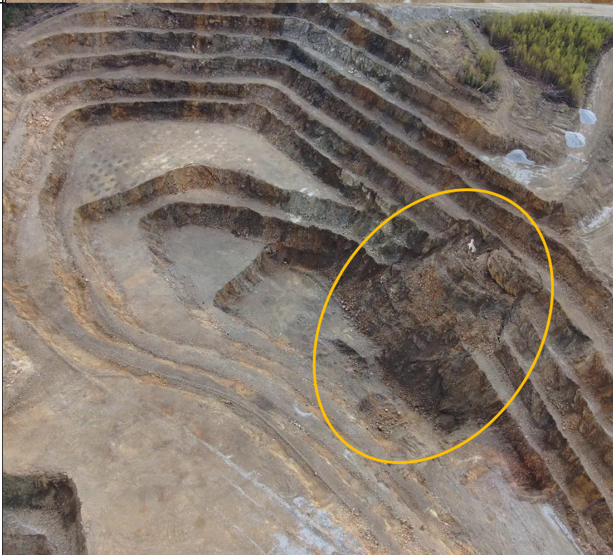
Photo 10: SE Sourdough Pit instability across several benches along the southwestern wall.
