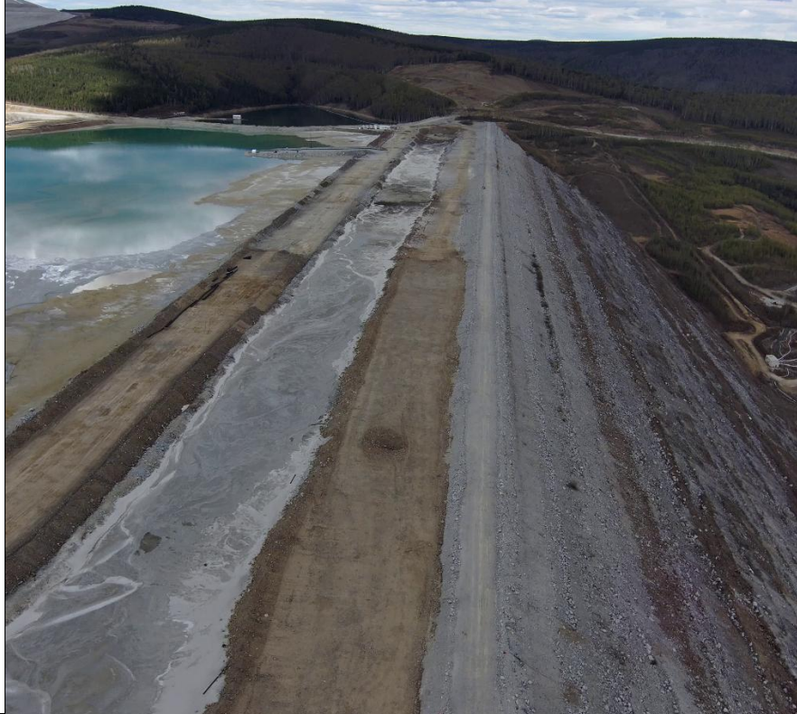
Photo 30: Northern view of the TSF Dam crest and face, north pond, and barge pond.
