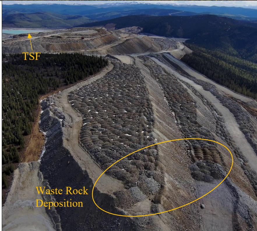
Photo 12: Active deposition of waste rock on the Victoria WRD, foreground.
