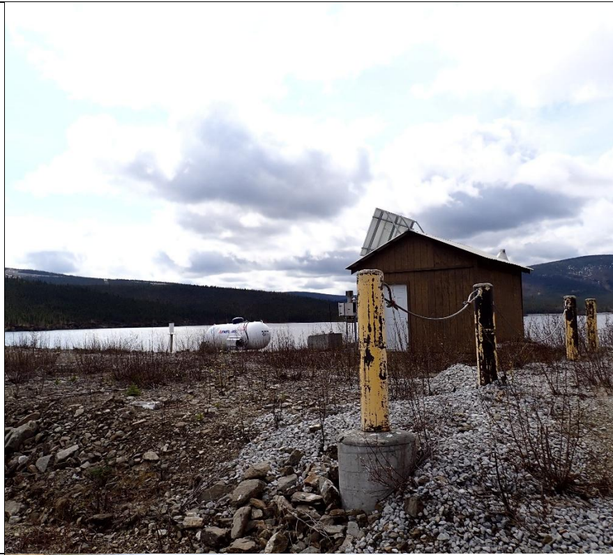
Photo 23: Fresh Water Reservoir valve house located on the northern end of the dam.
