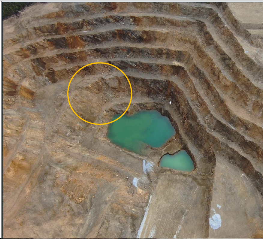
Photo 9: Ponding water observed in NE Sourdough Pit with minor in-pit instability.
