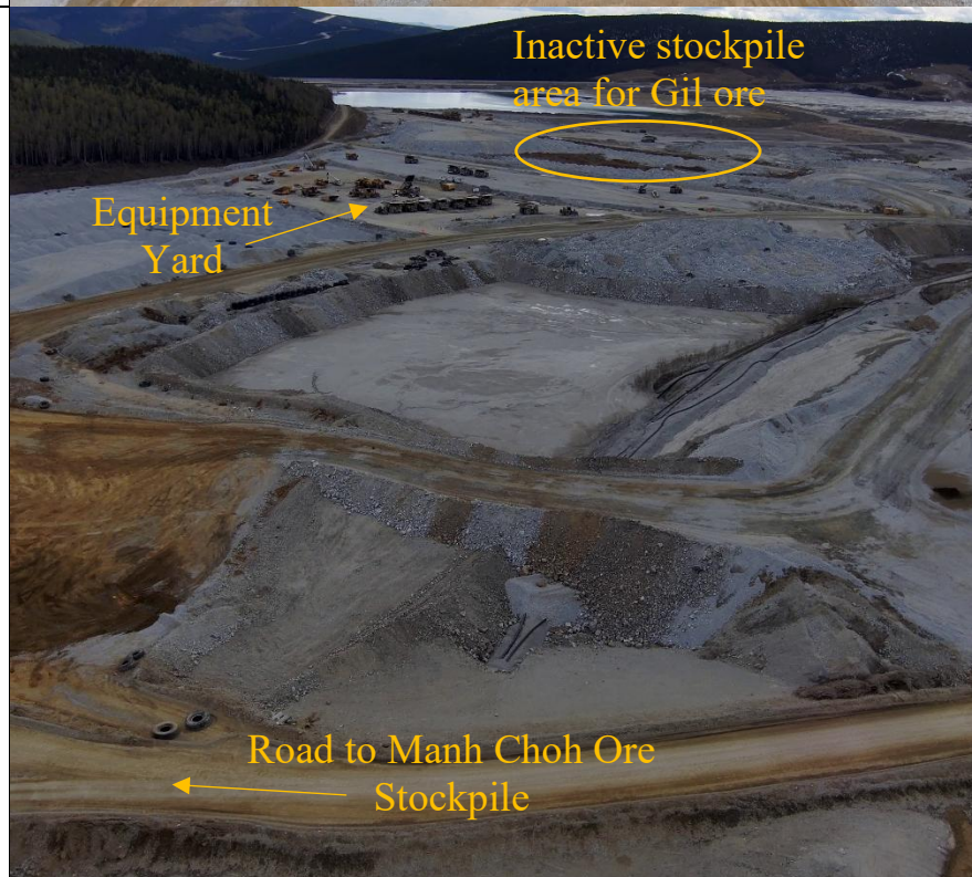
Photo 22: Overview of Central TSF comprised of areas of coarse tailings deposition, equipment yard, and ore stockpiles.
