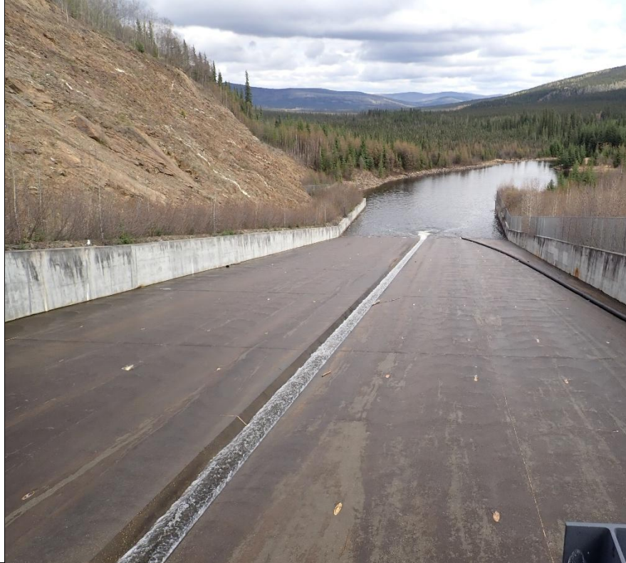
Photo 24: Water flowing across the length of the Fresh Water Reservoir Spillway.
