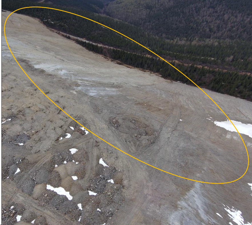
Photo 16: Final grading of benches along the western extent of Barnes Creek WRD.
