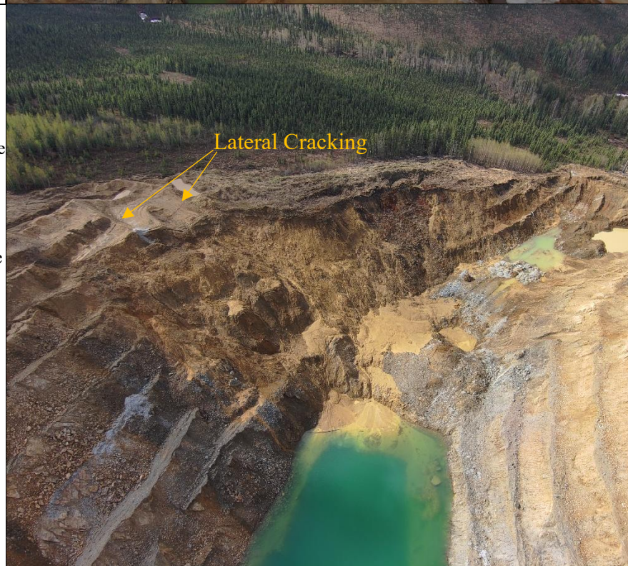
Photo 6: Main Gil pit wall instability west end on southern high wall. Material movement crosses all bench cuts.
