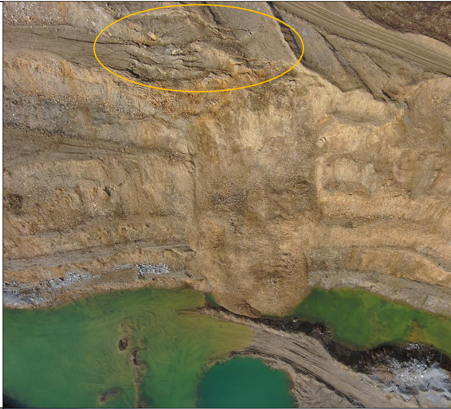
Photo 7: Material instability on the east end of the Main Gil pit northern high wall extending through all benches.
