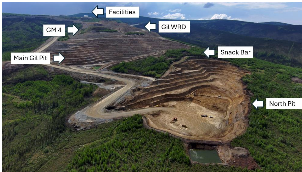
Photo 11: Gil Satellite Mine – Main Gil area with view of Facilities, Gil Waste Rock Dump (WRD), Growth Media Stockpile 4 (GM), Snack bar, and both the Main Gil and North pits. The view is to the south-southwest.
