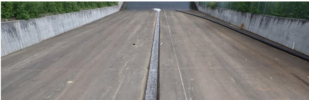
Photo 15: Fresh Water Reservoir Spillway.
