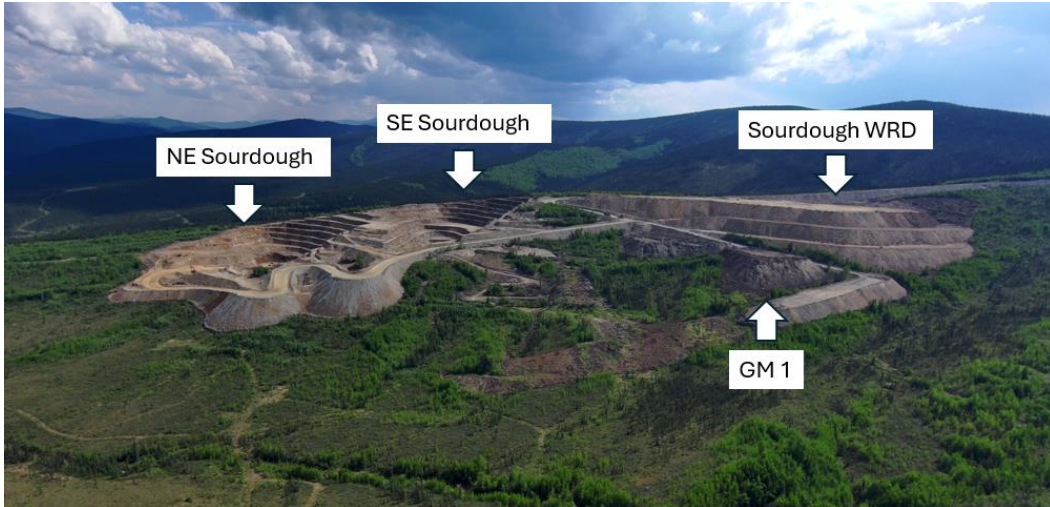
Photo 4: Gil Satellite Mine – Sourdough Ridge Area with view of NE and SE Sourdough pits, Sourdough Waste Rock Dump (WRD), and Growth Media (GM) Stockpile 1. The view is to the east-southeast.
