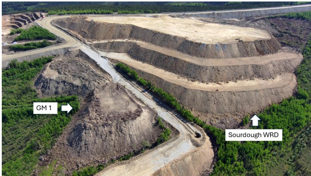
Photo 9: Gil Satellite Mine – Sourdough Waste Rock Dump (WRD) and Growth Media Stockpile 1 (GM). The view is to the east-southeast.
