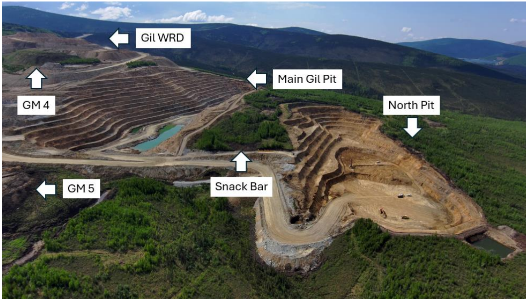
Photo 13: Gil Satellite Mine – Main Gil area with view of Gil Waste Rock Dump (WRD), Growth Media Stockpile 4 (GM), Main Gil Pit, Snack Bar, and southern edge of North Pit. The view is to the south-southwest.
