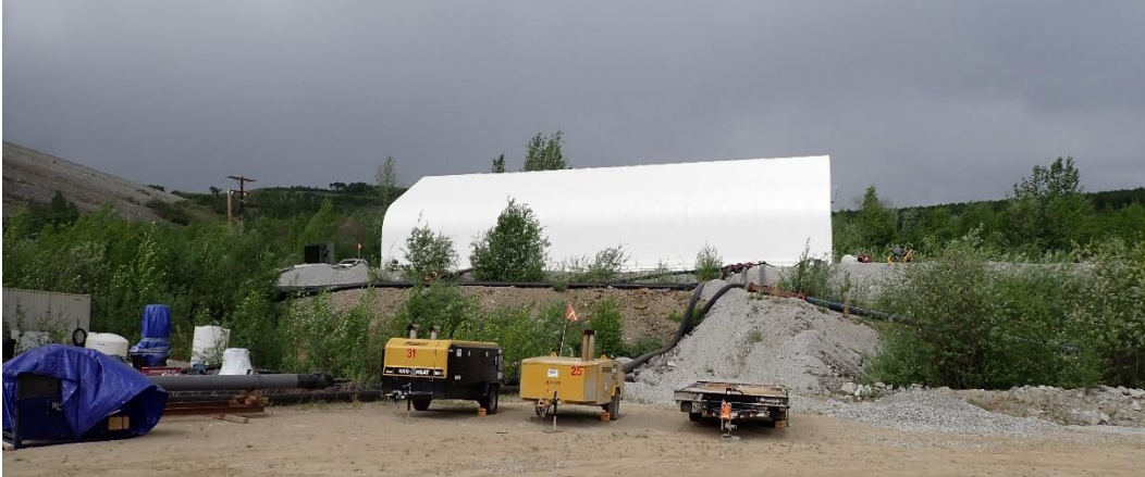
Photo 16: RO2. RO2 treats seepage and intercept water from the Tailings Storage Facility (TSF).
