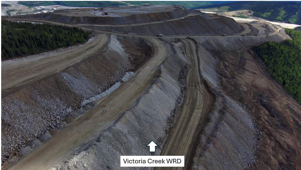
Photo 18: Victoria Creek Waste Rock Dump. Note the active mine trucks on the WRD. The view is to the east.
