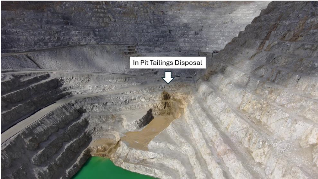
Photo 22: In Pit Tailings Disposal. The view is to the west.
