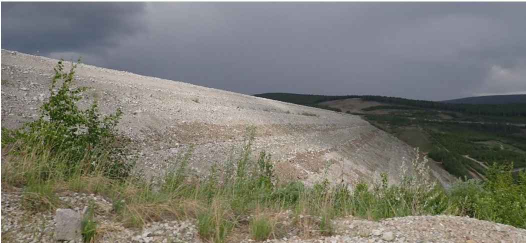
Photo 17: TSF Impoundment Dam. The TSF consists of tailings, decant pond, dam, causeways, seepage interception system, and seepage monitoring system. The tailings depositional area is within the Fish Creek drainage and includes portions of the Walter Creek, Pearl Creek and Yellow Pup drainages.
