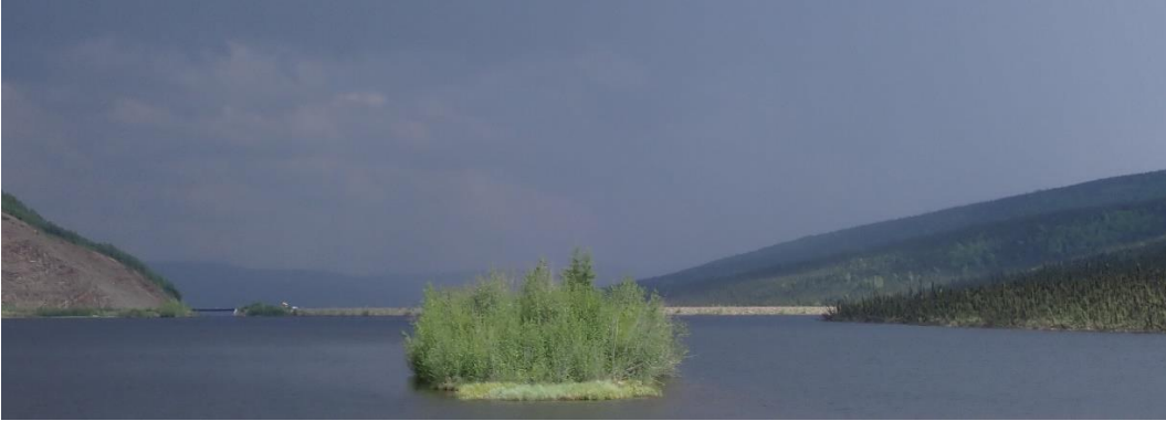
Photo 14: Fresh Water Reservoir.
