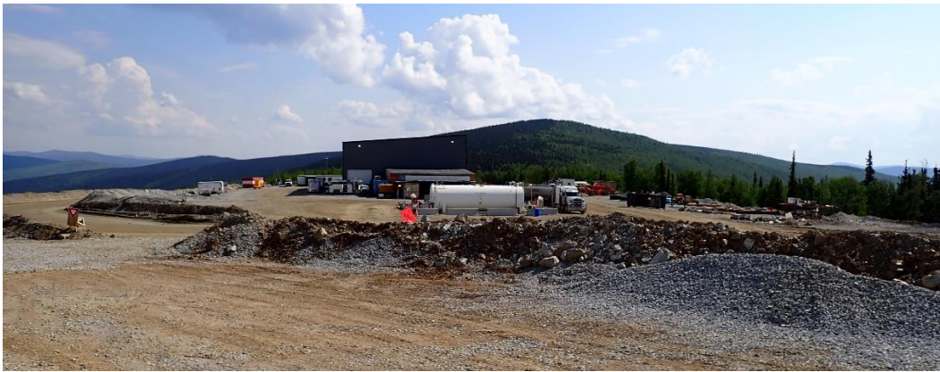
Photo 3: Gil fuel island, shop, and laydown area.
