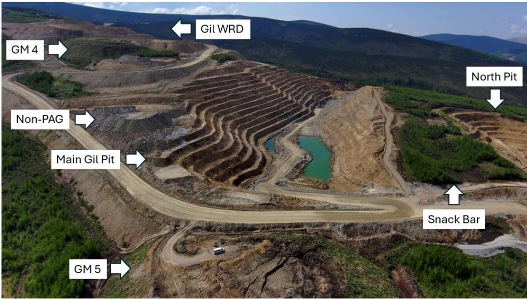
Photo 12: Gil Satellite Mine – Main Gil area with view of Gil Waste Rock Dump (WRD), Growth Media Stockpile 4 (GM), Main Gil Pit, Snack Bar, and southern edge of North Pit. The view is to the south-southwest.
