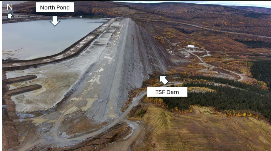
Photo 16: Northern view of the TSF Dam and North Pond . RO2 at the base of the dam. Note the new construction on the Pearl Creek Causeway (PCC).
