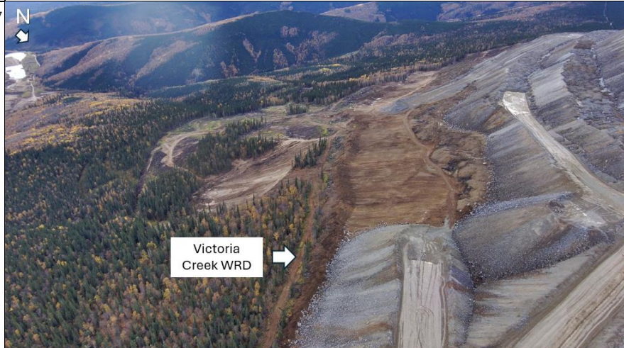
Photo 21: Southwest view of VCWRD including cleared area and areas of deposition.
