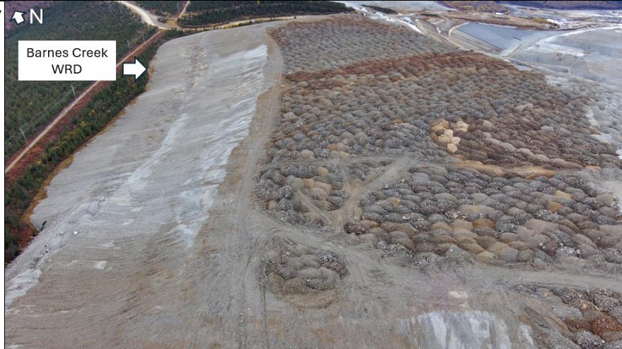
Photo 5: A northeast view of the northwest side of the BCWRD exhibiting final upper layer of deposition and initial phases of reclamation (contouring) .
