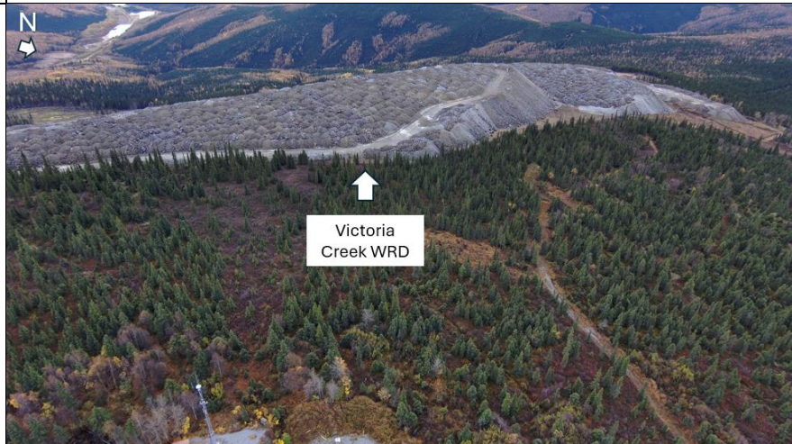
Photo 24: West view of the VCWRD.
