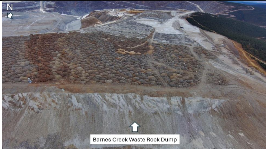
Photo 6: Another view of the north west side of the BCWRD showing final deposition and initial phases of reclamation (contouring).
