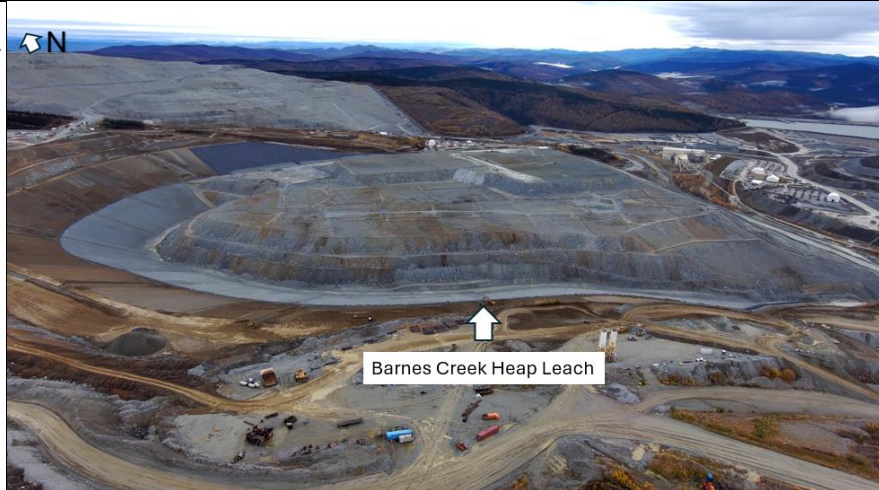
Photo 3: Another view of the BCHL . WCHL upper left.
