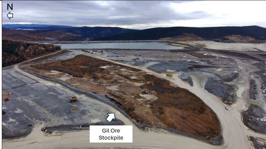
Photo 15: Another view of the GOS . TSF north and south ponds in background.
