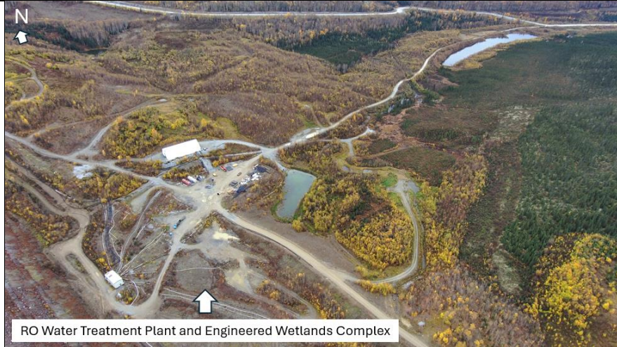
Photo 19: RO2 and engineered wetlands complex below the TSF Dam.
