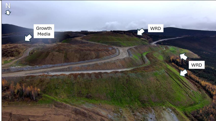
Photo 33: Main Gil GM 4 and GWRD . Note the hydroseeding taking hold on the GWRD.
