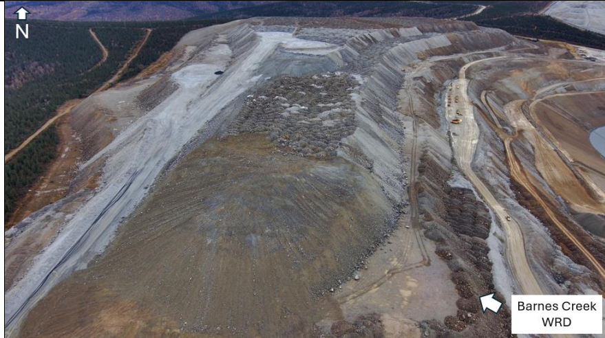
Photo 7: Initial phases of reclamation at the southern end of the BCWRD.
