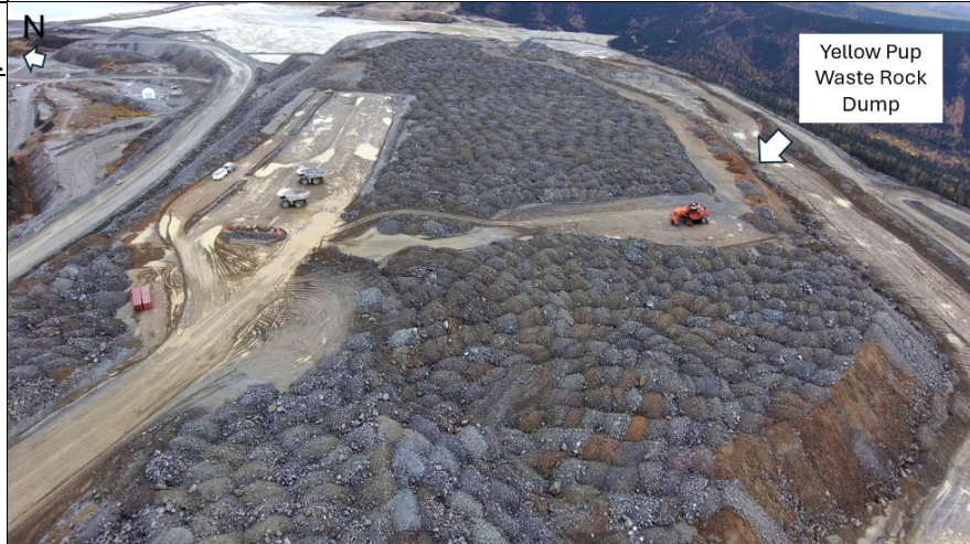
Photo 26: Easterly view of the top of the YPWRD.
