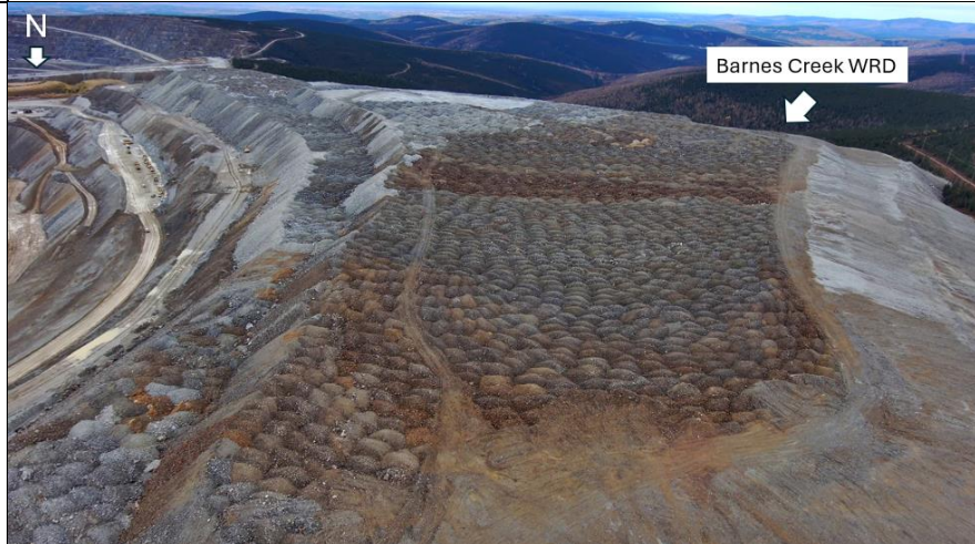
Photo 4: Barnes Creek Waste Rock Dump (BCWRD) . Southerly view of the top, final deposition of tailings and initial reclamation phase (contouring) of the west and northwest sides.
