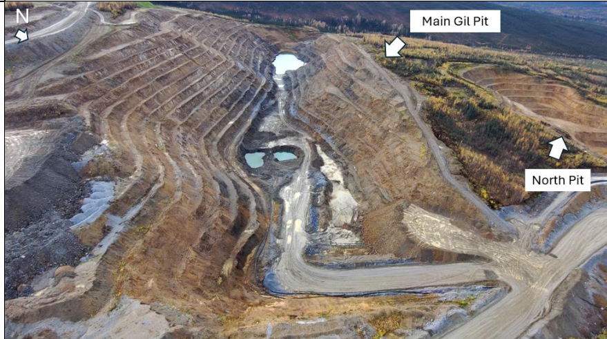
Photo 28: Main Gil Pit , Snack Bar and North Pit to the right.
