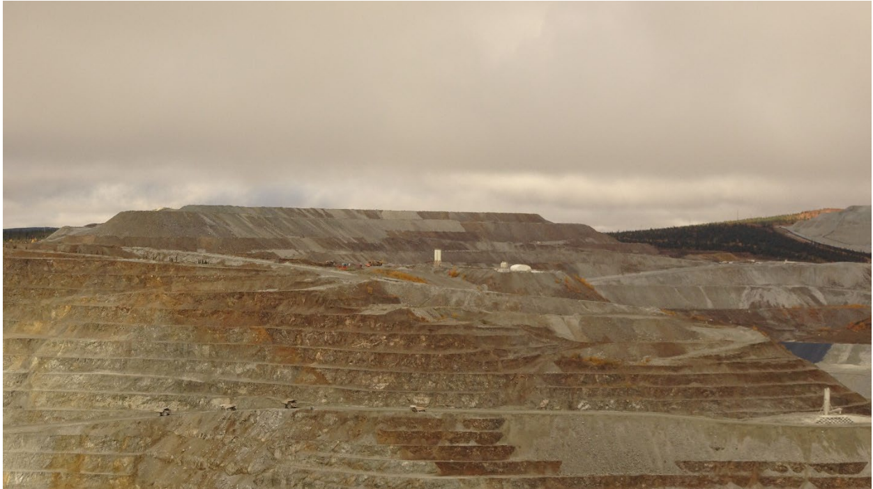
Start of regrading on Northern edge of Barnes Creek WRD
