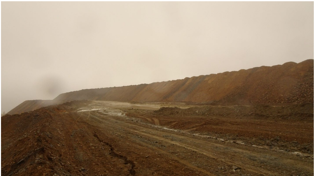
Settling crack on waste rock dump at Gil Extension
