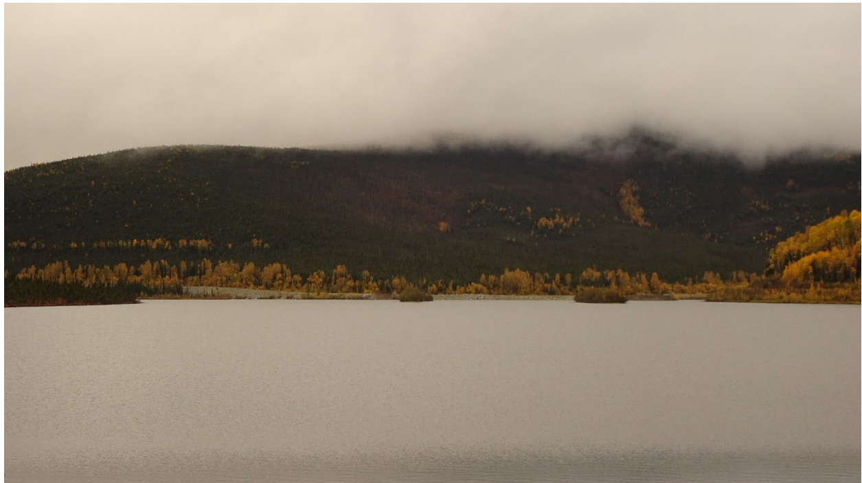
Freshwater Reservoir from dam.
