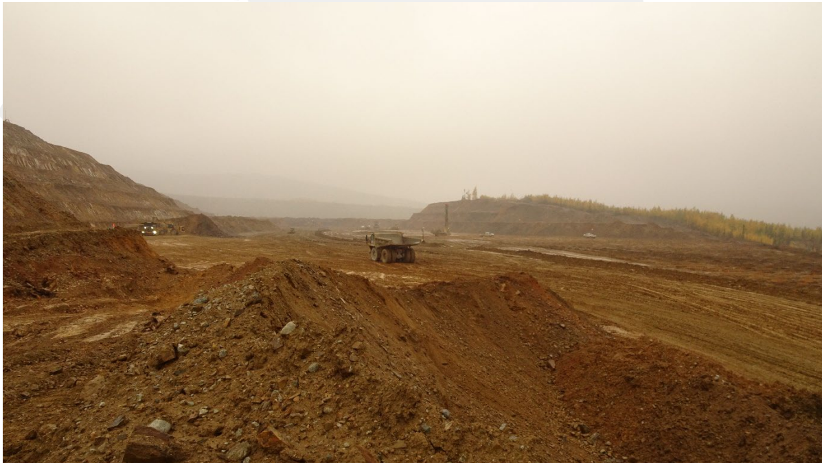
Bottom of main pit at the Gil Extension.
