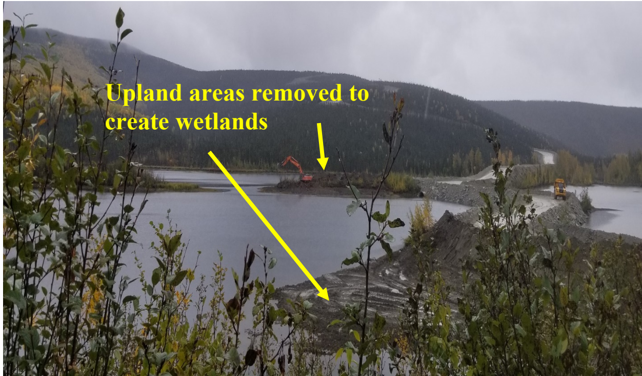
Figure 3. Two upland areas removed during low water to create aquatic habitat in the WSR. These lowland areas were flooded when WSR water levels returned to normal on September 16, 2022.
