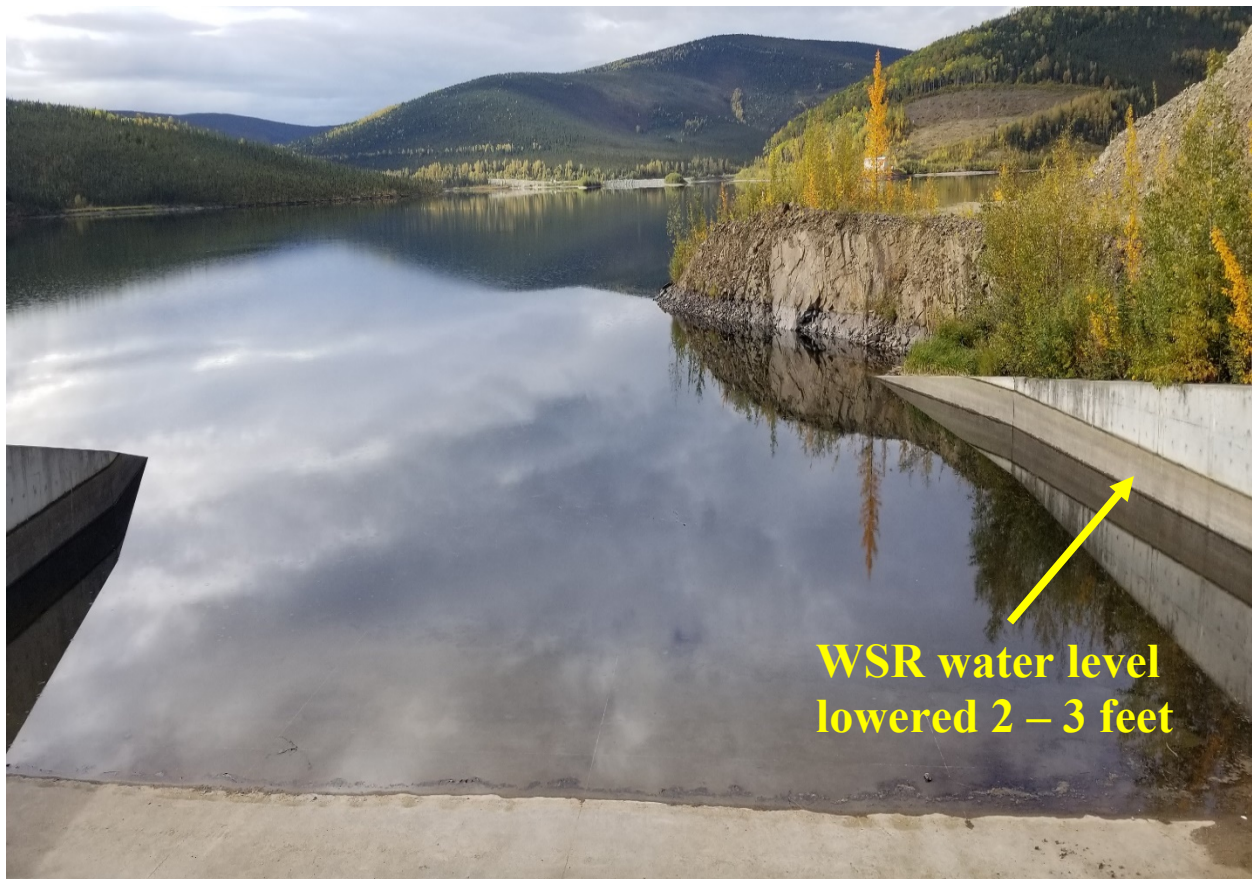
Figure 2. WSR lowered 2 – 3 vertical feet for spillway inspection and maintenance, September 6, 2022.
