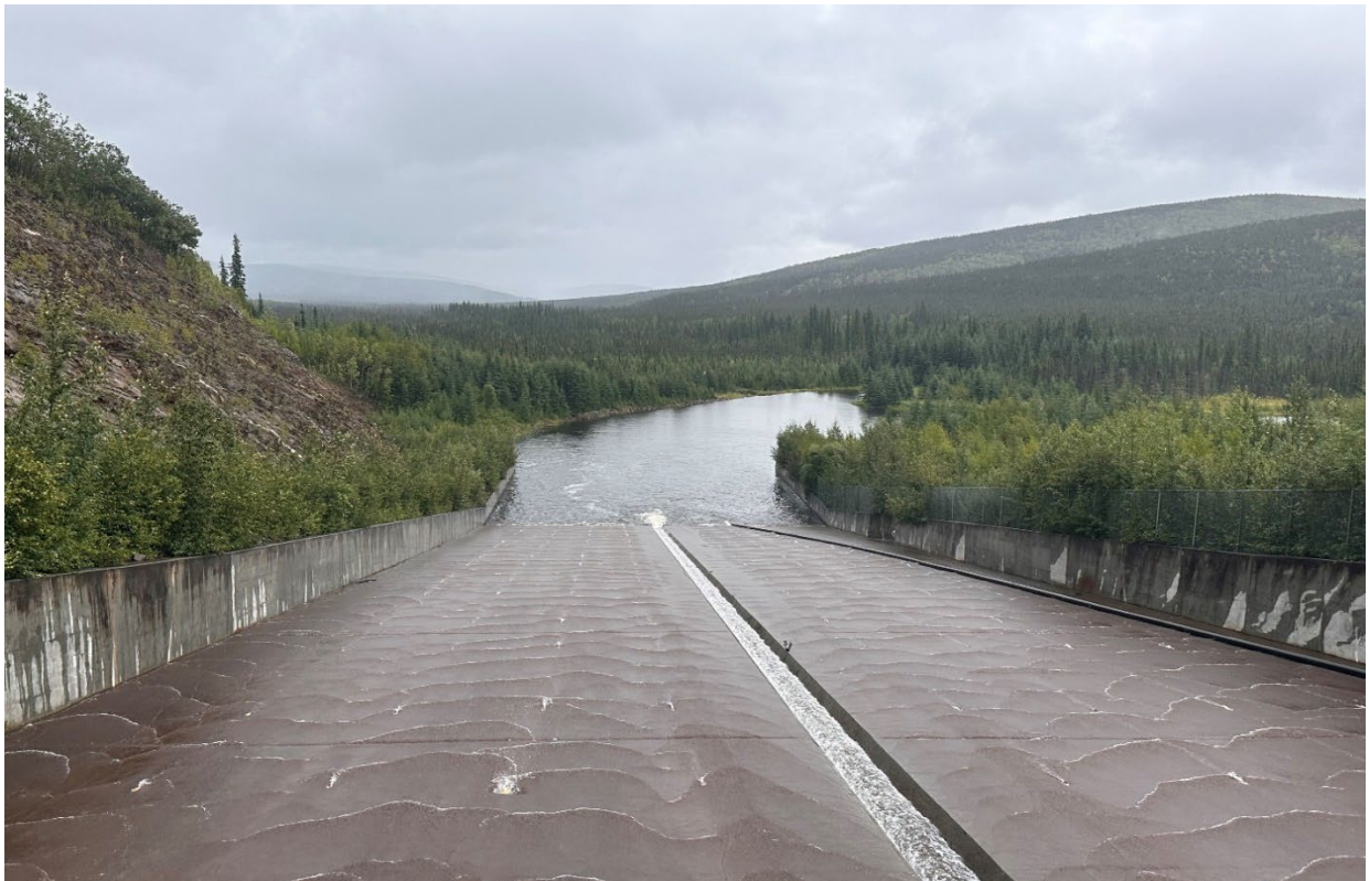
Figure 1. Water Supply Reservoir spillway leading to the Stilling Basin, August 2, 2024.
