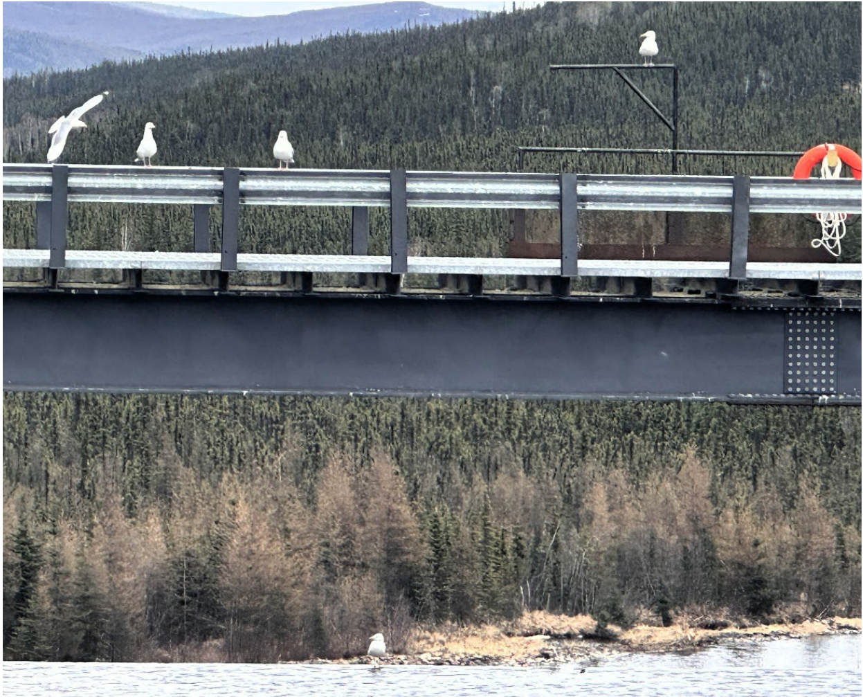
Figure 22.— Gulls observed on the WSR Spillway bridge, May 2026.
