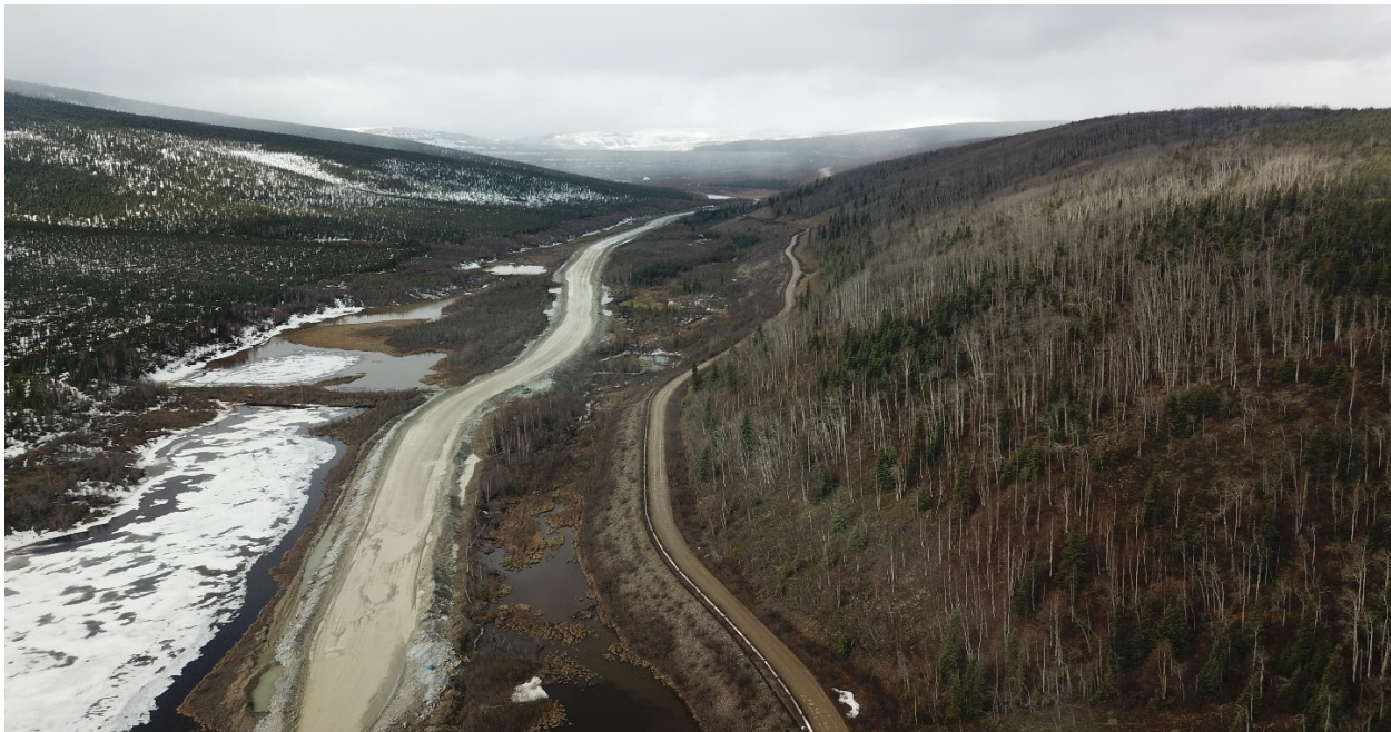
Figure 2. Centerline Road widened and improved during 2021 and 2022.
