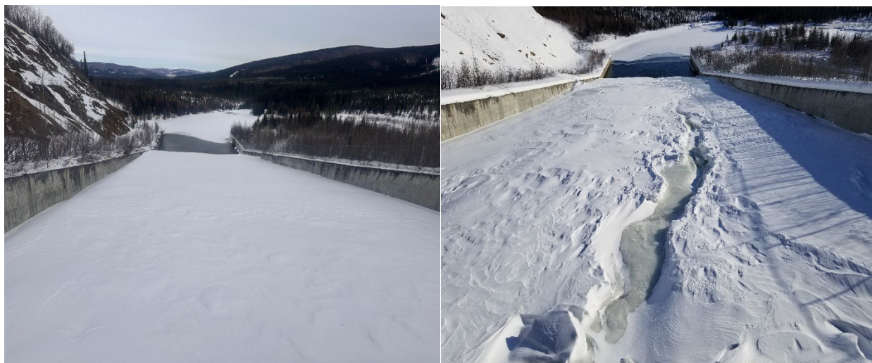
Figure 5.—Fort Knox WSR Spillway, April 22, 2026 (left) and March 31, 2020 (right).
