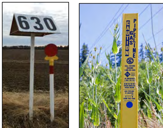
Figure 8 – Typical line markers: Aerial mile markers (left) and “Warning Buried Pipeline” marker (right).
