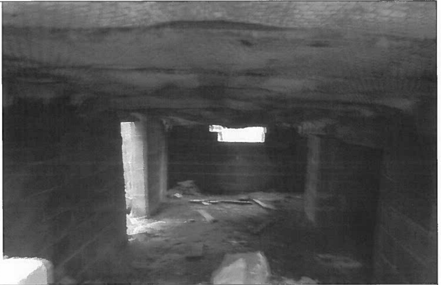
Crawlspace of block structure on Lot 12
