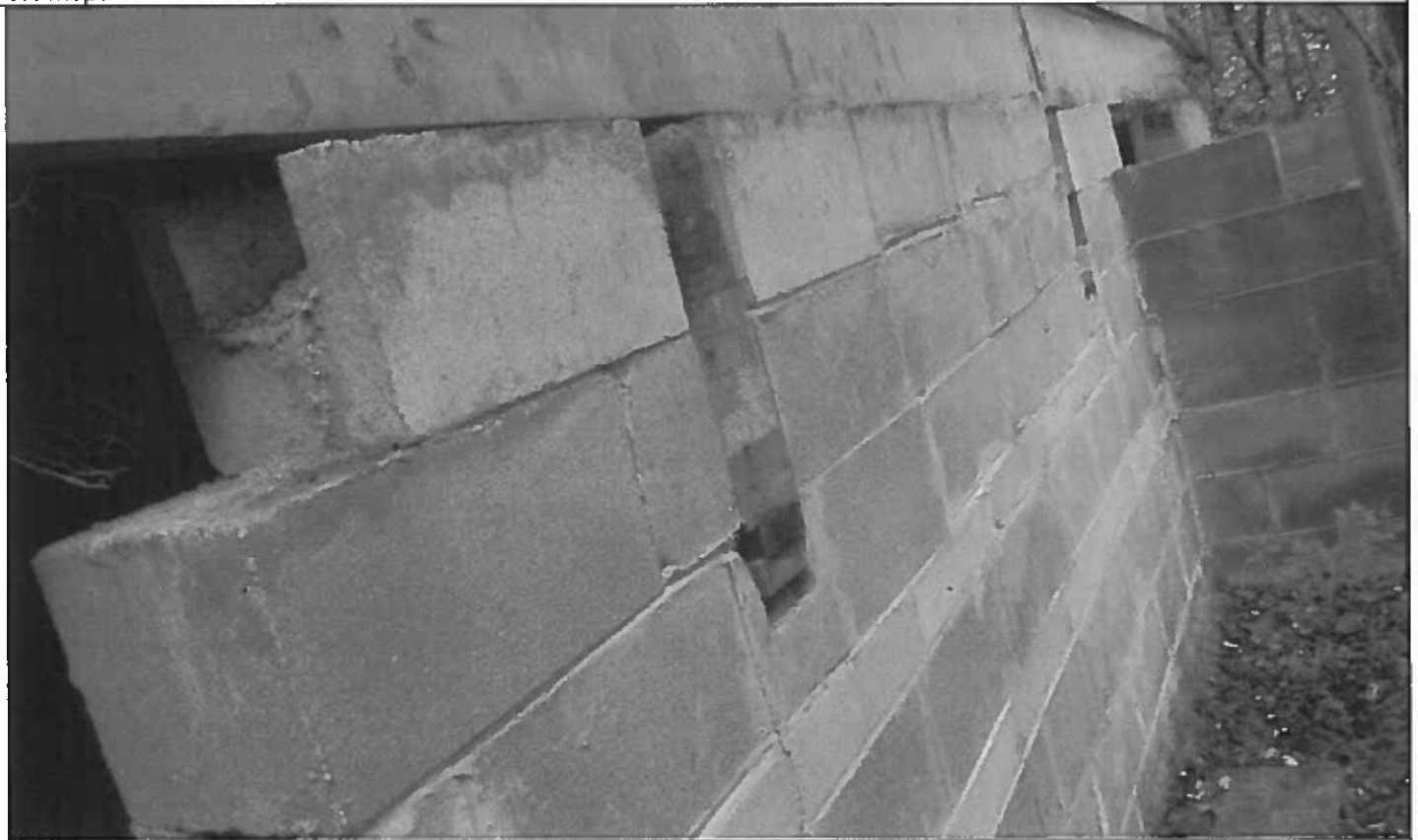
Block structure on Lot 12
