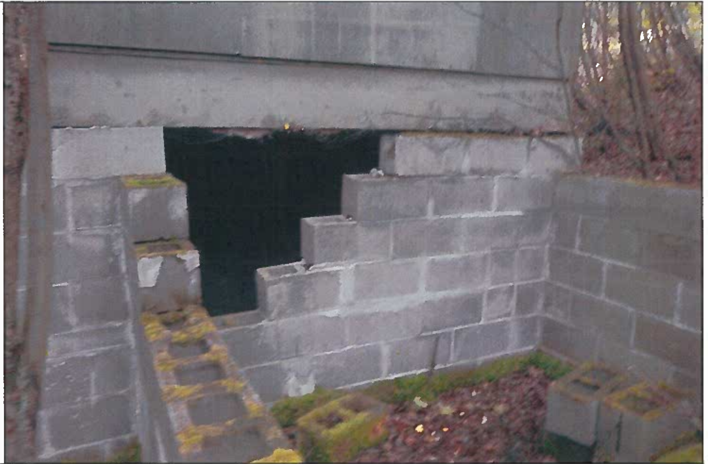
Block structure on Lot 12
