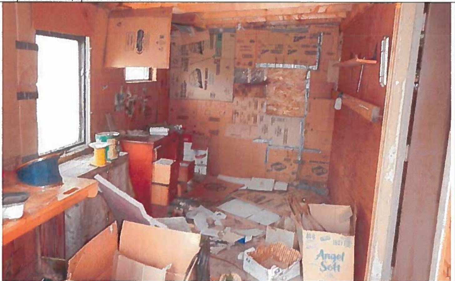
Interior of lean-to
