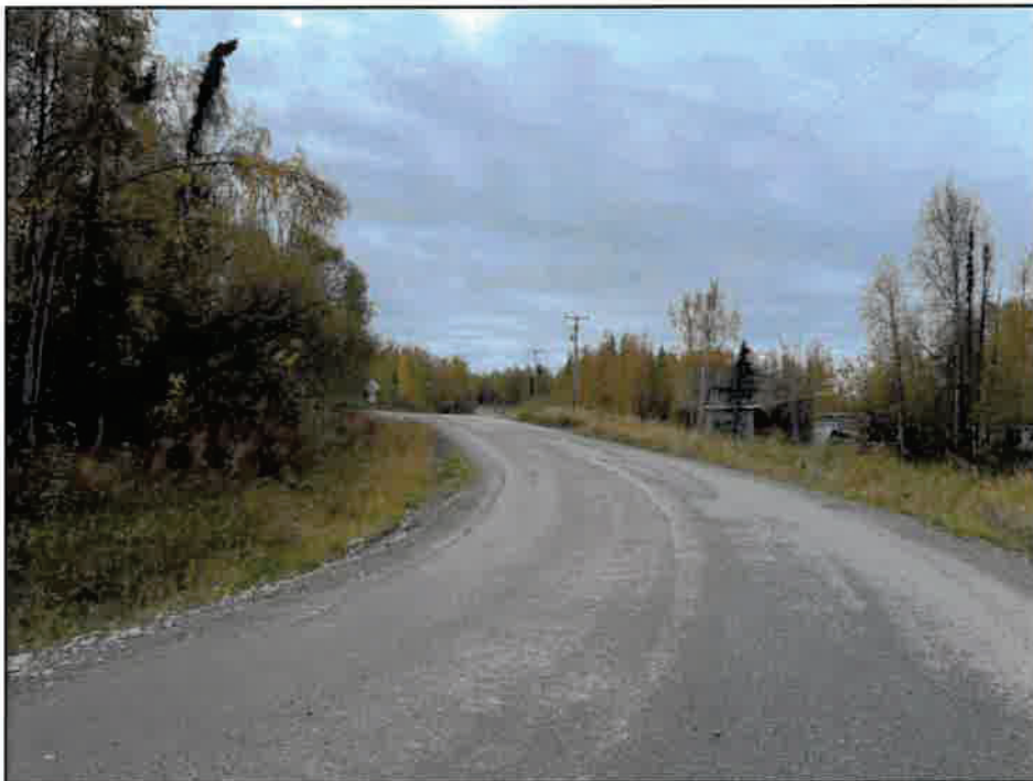
Looking south down North Windy Bottom Road.
