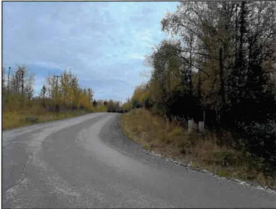
Looking east down North Windy Bottom Road.
