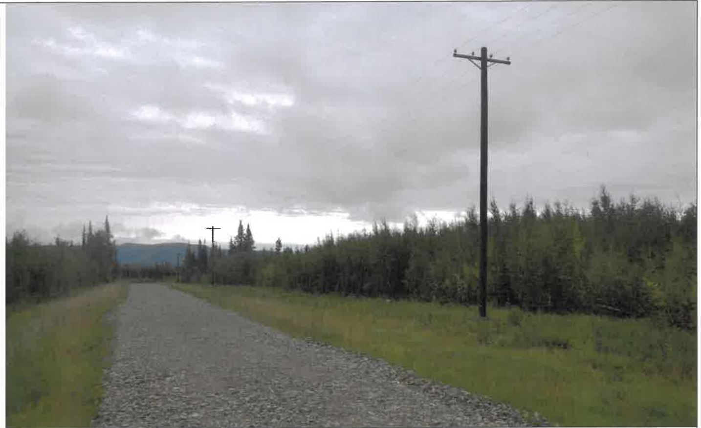
Access along Kohlrabi Court.
