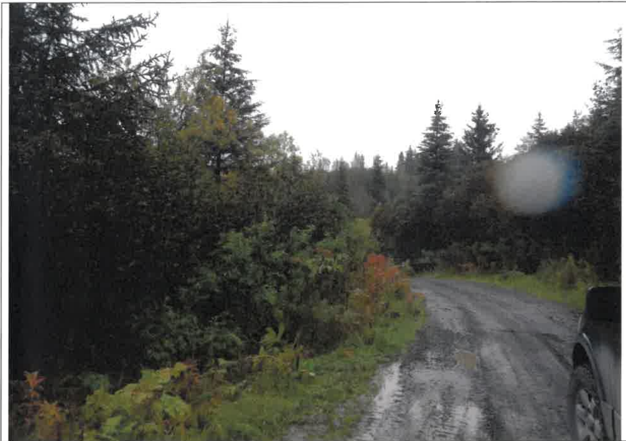
Wagon Road diminishes in quality prior to Lot 1 Block 5.
