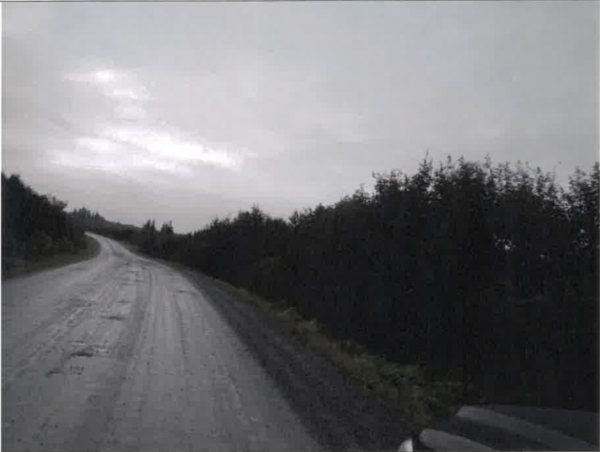
Access to ADL 234465, looking south.
