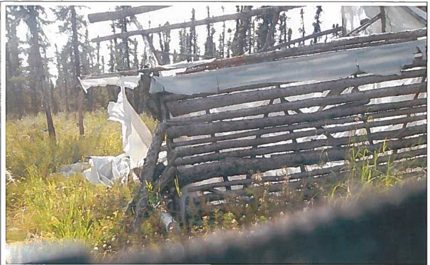
ADL421038. Debris on parcel.
