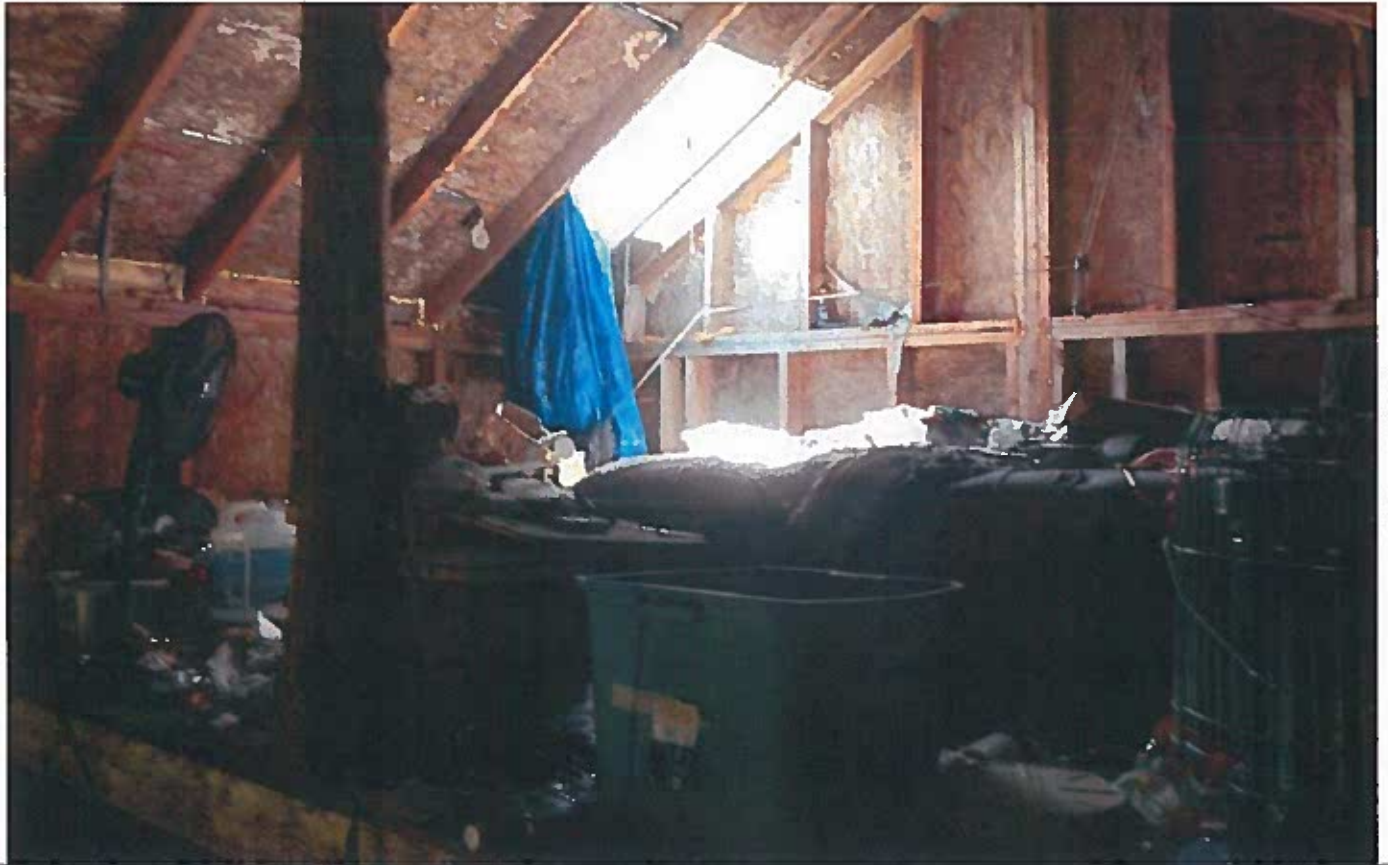
Loft. Open to weather.
