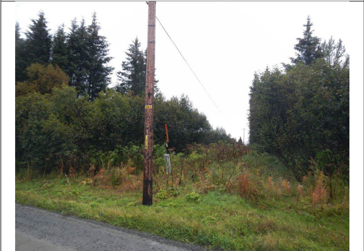
Lot 3 Block 1. Near southern lot line. Overhead power on site.
