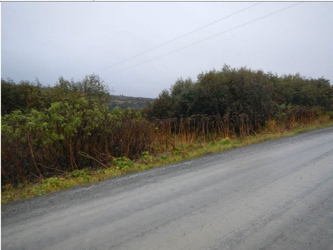
Lot 1 Block 4. Overhead power lines near southern lot line.
