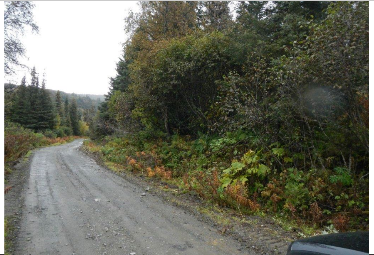
Lot 1 Block 4. Secondary access along Wagon Road.
