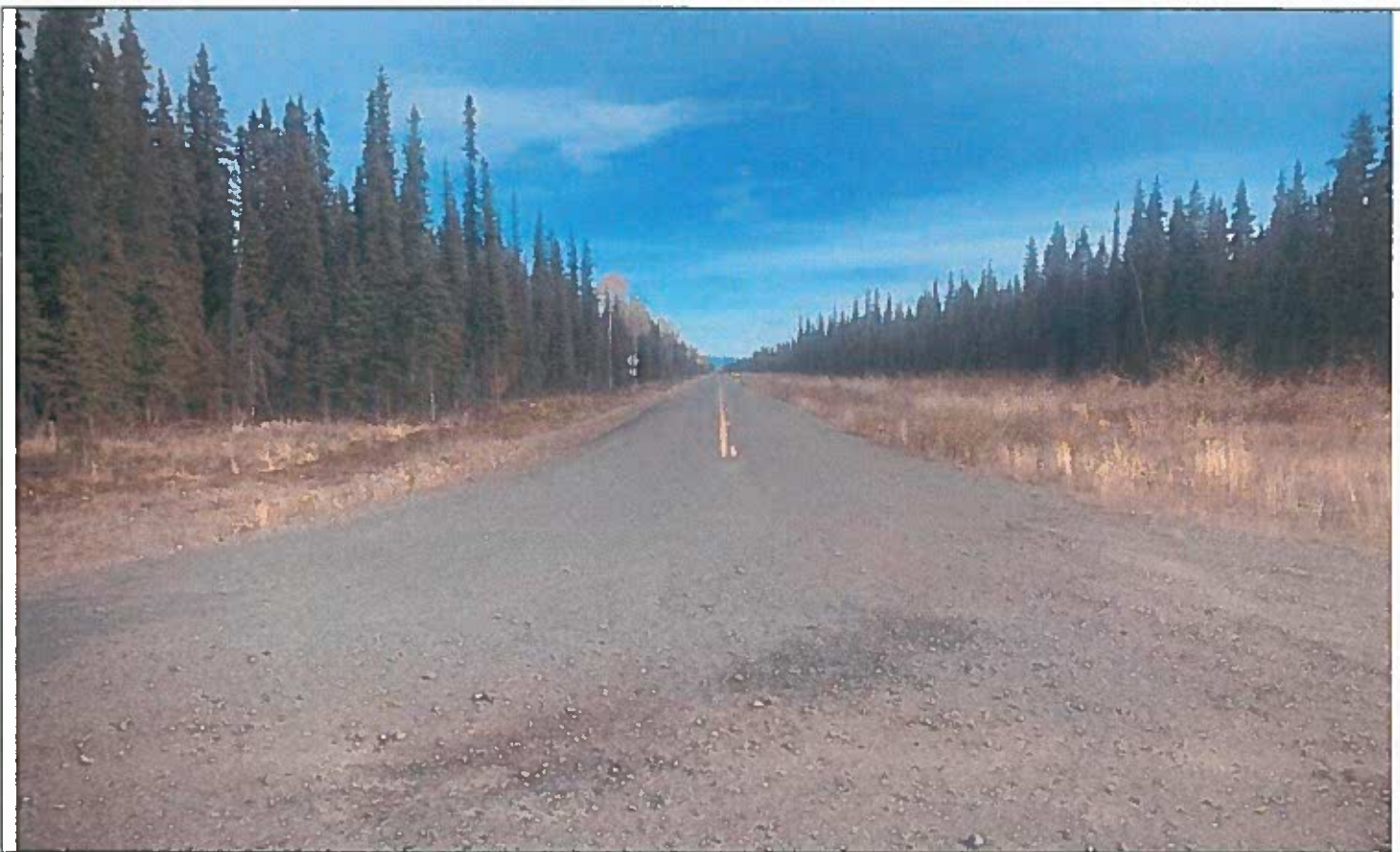
Borealis at Northwest corner of subdivision. Lots 10, 11, 12 & 1, Block 4 on right (Surveyor Photo).
