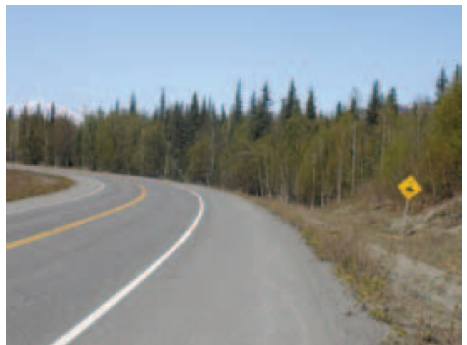
7D. Trail crossing at MP 130
