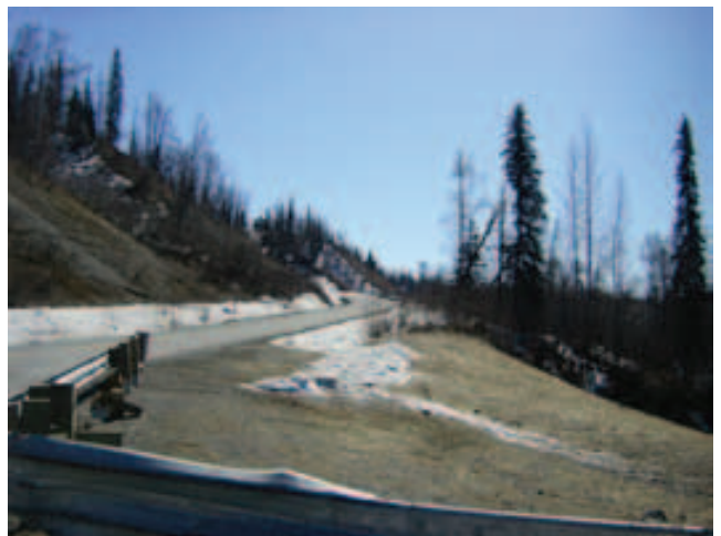
8D. Exiting the Chulitna Bridge
