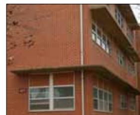
**Visor Roof**—Narrow roof segments cantilevered from the wall.
