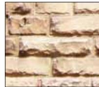
**Rustification**—The treatment of stone masonry that deeply cuts back the joints between the blocks. The surfaces of the blocks may be smoothly dressed, textured, or extremely rough or quarry-faced.
