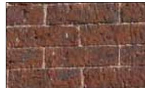
**Bond**—The laying of bricks or stones regularly in a wall according to a recognized pattern for strength. Masonry bond is essential to brickwork when wire reinforcement is not used.
