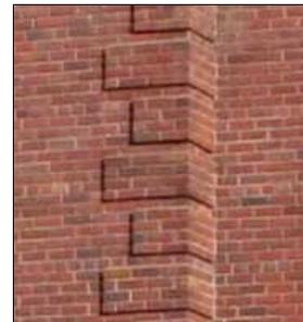
**Quoins**—Heavy blocks, generally of stone or wood, cut in emulation of stone, and used at the corners of buildings to reinforce and ornament masonry walls, or used in wood as a decorative feature only.
