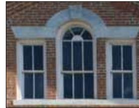
**Palladian Window**—A window design featuring a central arch opening flanked by lower, square-headed openings separated by columns, pilasters, piers, or narrow vertical panels.
