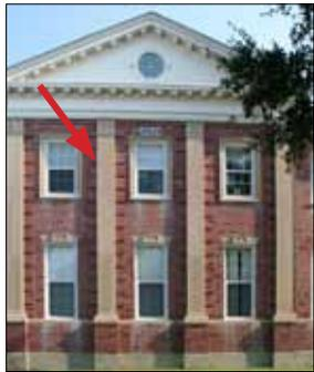
**Pilaster**—A flat-faced representation of a column, projecting from a wall.
