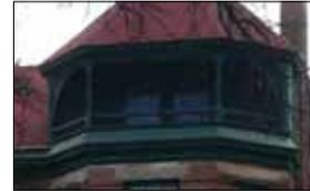
**Engaged Porch**—A porch whose roof is continuous structurally with that of the main section of the building.
