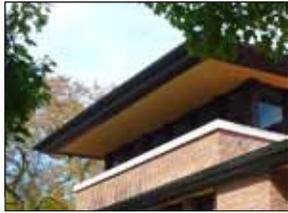
**Cantilever**—A bracket or horizontal beam that is only anchored at one end that supports a part of a building, a balcony or a roof.
