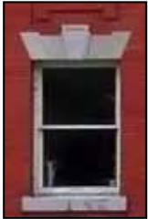
**Flat Arch**—An arch formed on a straight horizontal plane; also referred to as a jack arch.
