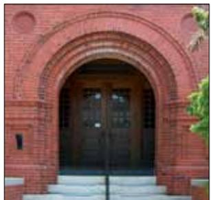
**Arch**—A structure formed of wedge-shaped stones, bricks, or other objects laid so as to maintain one another firmly in position.
