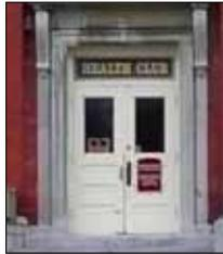
**Half-glazed Door**—A door consisting of glass for half of the surface, typically the upper half, with wood panel or panels below.
