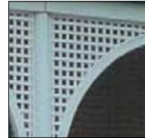
**Lattice**—A network, often diagonal, of interlocking lath or other thin strips, used as screening, especially in the base of a porch.
