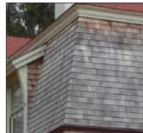
**Mansard Roof**—A modification of the hip roof in which each side has two planes, the upper being more shallow; see *Roof*.
