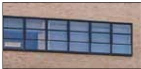
**Ribbon**—One of a horizontal series of three windows or more, separated only by mullions, that forms a horizontal band across the facade of a building.
