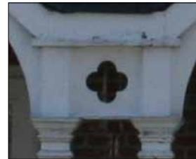
**Quatrefoil**—A round pattern, sometimes in a window or vent, which is composed of four equal lobes, like a four-petaled flower.
