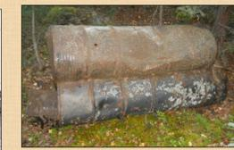
Figure 17. Four drums (1941-42) welded together to form an expedient water heater at a road construction camp (1940s).
