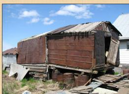
Figure 20. Drums used as building support piers, and sheathing for siding and roofing (2010).
