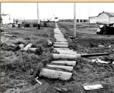
Figure 21. A tundra walkway through a village consisting of a linear series of drums (1970s).
