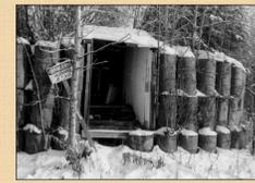
Figure 18. Cold War era anti-aircraft building buttressed with soil-filled drums (1950s). (Brian Allen photo).
