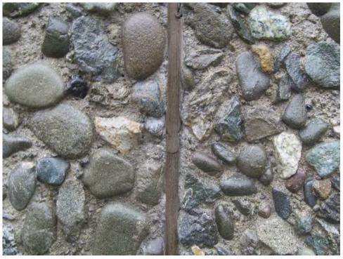
Figure 44. Exposed aggregate wall with pebble dash (source: TNSDS 2014).
