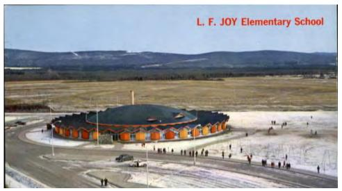
Figure 42. Joy Elementary, Fairbanks, 1962; displays folded concrete plate technology along the edges of the domed roof. Post Card caption reads" L. F. Joy Elementary School. One of the buildings in the Fairbanks, Alaska modern School system. Recipient of national and international recognition for architectural design." (source: Mike Roberts, nd).
