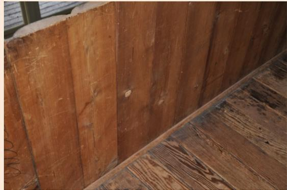
The loft pony wall is comprised of vertical cedar siding, found throughout the building. It is attached at the floor boards. Each piece of siding is attached by four nails. Quarter round finishes the wall on the loft side. Evidence that the pony wall is pulling away from its vertical orientation is seen near each wall. This attachment method creates an unstable wall and a safety concern.
