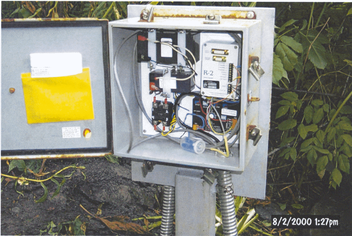
Photo 1: Instrument shelter with electronic data recorders.
