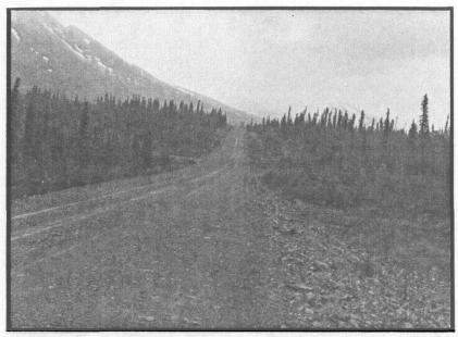
Uniformly wide cut strips prevent the road from blending with the landscape. Instead, the depth of the cut can be varied, allowing trees close to the road near the crest of the rise to frame the next view.
