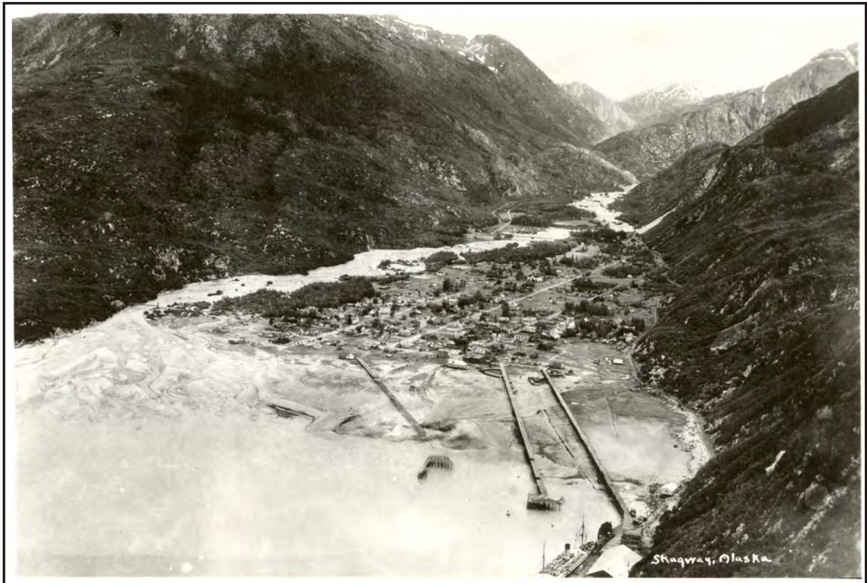
Figure 1. The town of Skagway, June 22, 1929. The Skagway River flows south into Taiya Inlet. Photo KLG0 SO49-949, Klondike Gold Rush National Park, Skagway.
