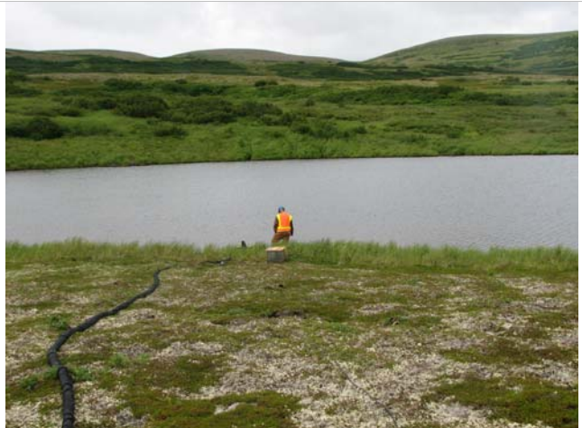
Figure 8. Water supply for drill rig 3.
