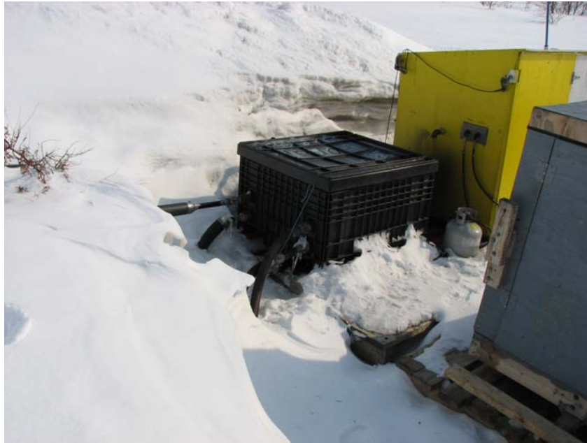
Figure 5. Circulation tank at water source location for rig no. 2
