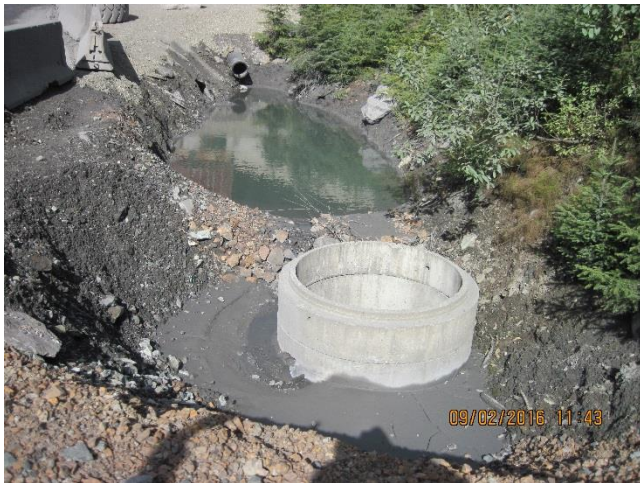
Photo 12. Rock check dam and sump across from DB-01.
