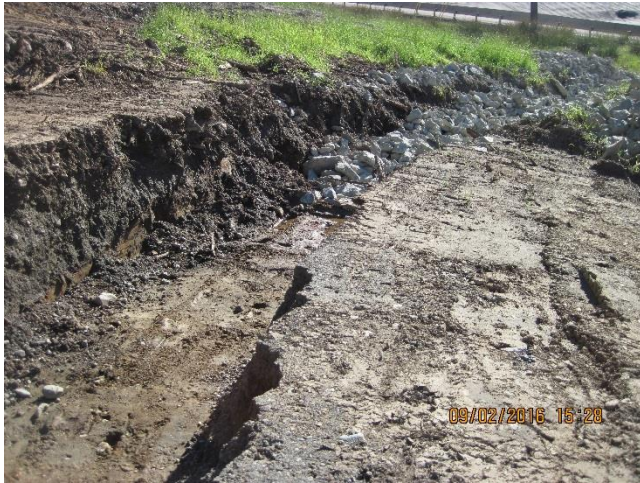
Photo 28. An up slope non-contact water diversion trench at the 0.9 mile B-road.
