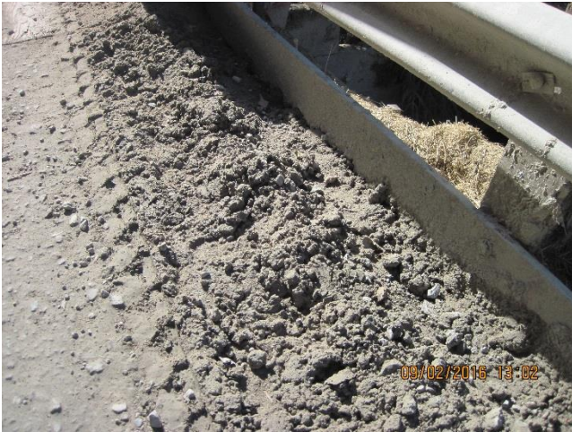
Photo 23. Temporary barrier at the downhill/streamside of Falls Creek Bridge.
