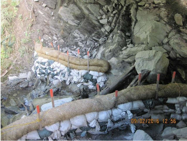
Photo 22. Sandbags and straw wattles placed below Falls Creek Bridge.
