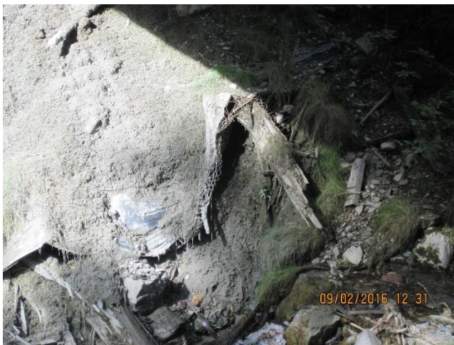
Photo 18. Downhill side of Killer Creek Bridge.
