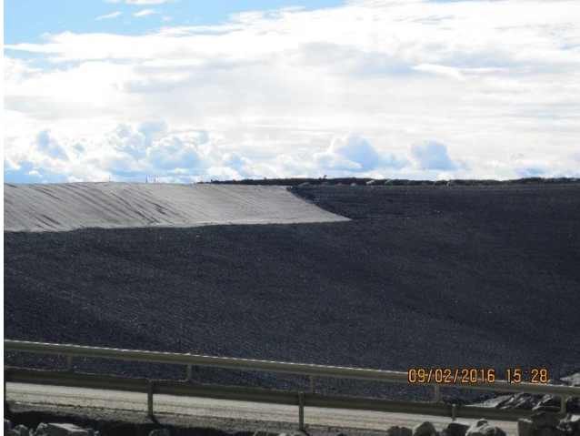
Figure 4. Class-1 waste rock and organic placed over tailing at the outer slopes.
