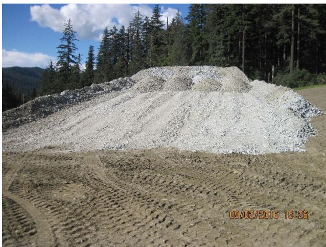
Figure 6. Crushed bedrock from the Pond-10 construction stockpiled at the 0.9 mile B-road.
