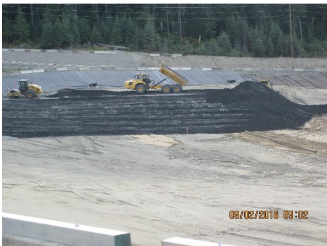
Photo 3. HGCMC continues to deposit tailings at the TDF expansion area.
