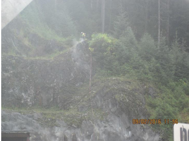
Photo 1. Rock bolting above the 920 portal.
