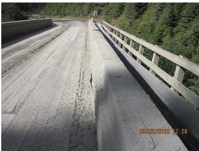
Photo 21. Sediment accumulation on the rails of Killer Creek Bridge.
