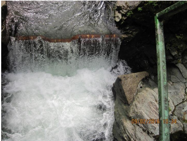
Photo 16. Upstream image shows 1 of 3 concrete steel capped weirs.
