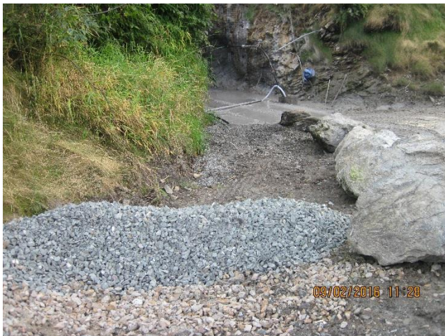
Photo 8. Imported rock covering the pipeline from the caisson to the 1350 adit.
