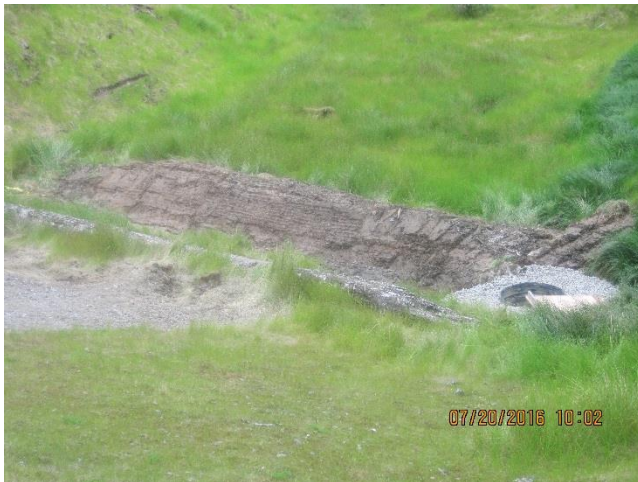
Photo 1. A trench installed at the 1350 area.
