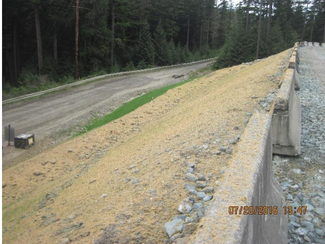
Photo 23. Berm for the Sand Pit has been hydroseeded.
