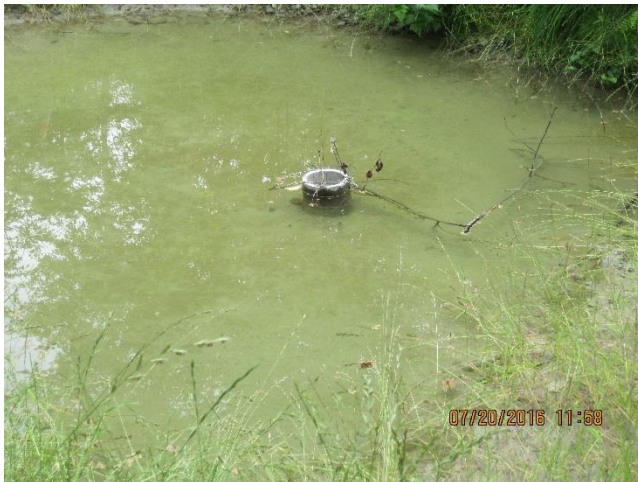
Photo 15. The BMP's stand pipe, sumps and rock check dams installed need to be frequently monitored and maintained.
