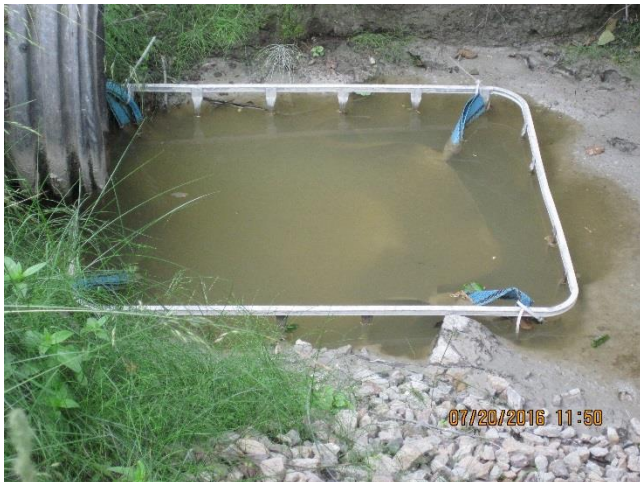
Photo 12. 3.1 mile B-road removable sediment screen.
