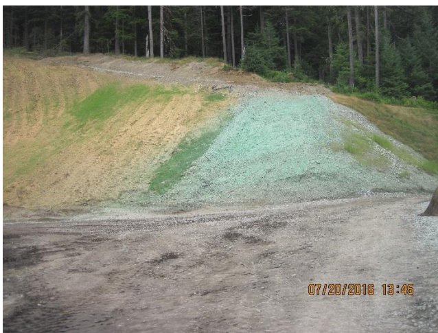
Photo 22. Hydroseeded area at the Sand Pit to prevent erosion.
