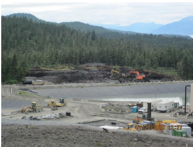
Photo 19. Excavators are removing organic material for the Pond-10 construction.
