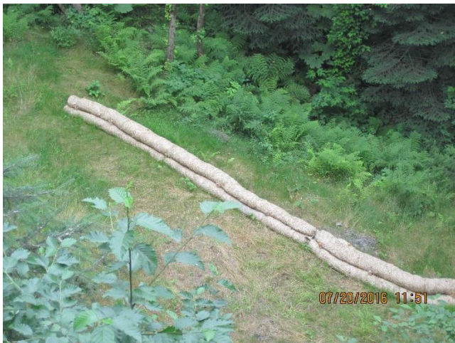
Photo 13. Straw wattles placed to capture sediments from stormwater runoff.
