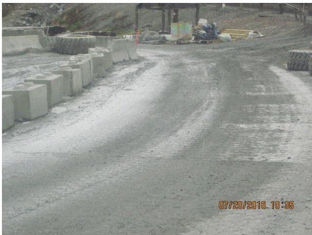
Photo 4. 920 concrete overlay has been repaired.
