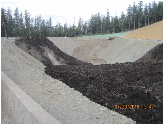
Photo 20. Excavated organic material from the Pond-10 construction.
