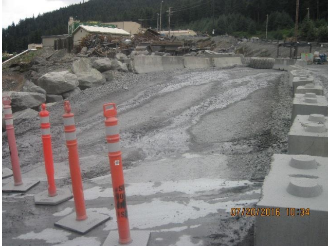
Photo 5. Image shows the area used for rerouting mine traffic.
