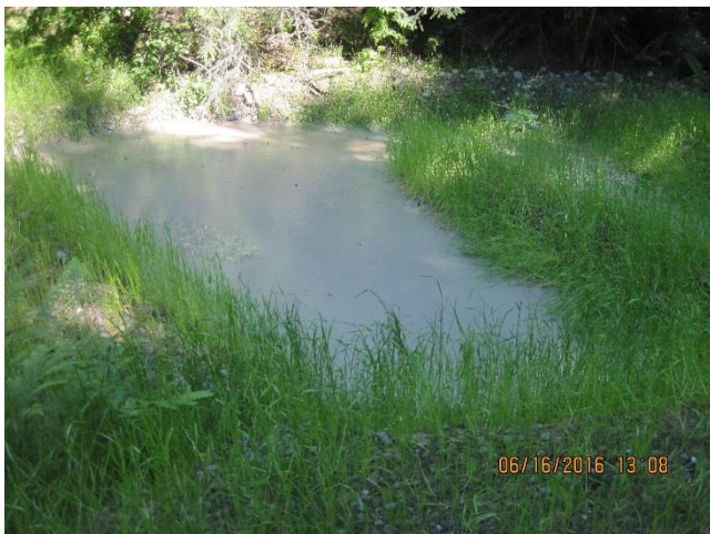
Photo 22. Zinc Creek Bridge sump.
