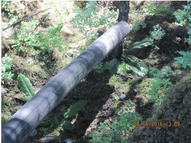
Photo 24. Zinc Creek Bridge standpipe drain.
