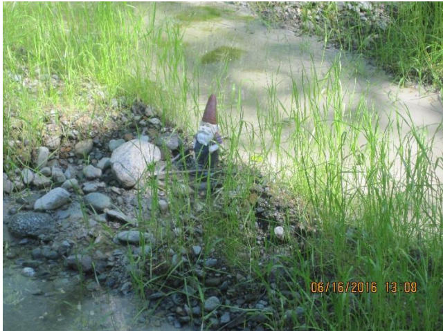
Photo 21. Zinc Creek Bridge rock check dam.
