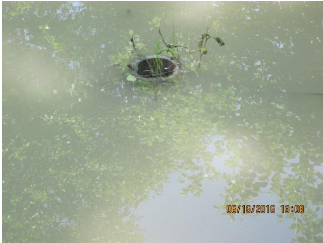
Photo 23. Zinc Creek Bridge standpipe.
