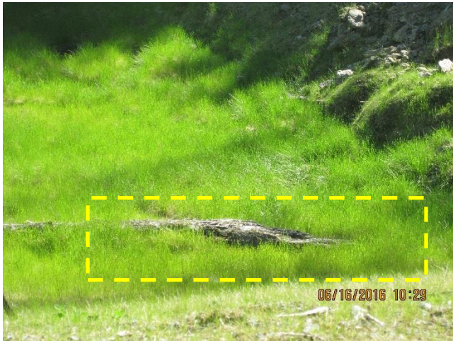
Photo 7. Possible location for a sump to divert water to the 1350 adit sump.
