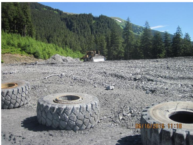
Photo 16. Bull dozer leveling an area for Class 1, 2, and 3 stockpiles.
