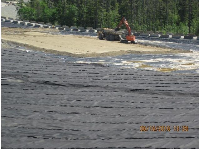
Photo 26. Service sand layer being placed over the geotextile.
