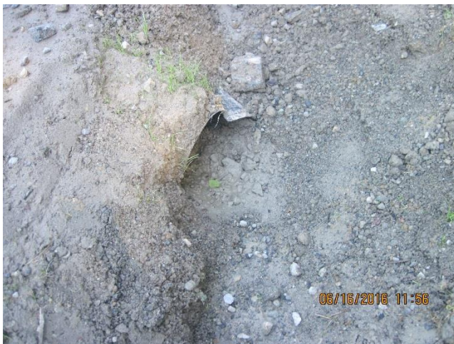
Photo 19. Nearby culvert has been mucked.
