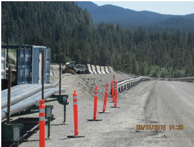
Photo 33. 1.0 mile B-road realignment.
