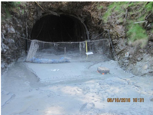
Photo 5. 1350 adit sump is mucked when necessary.
