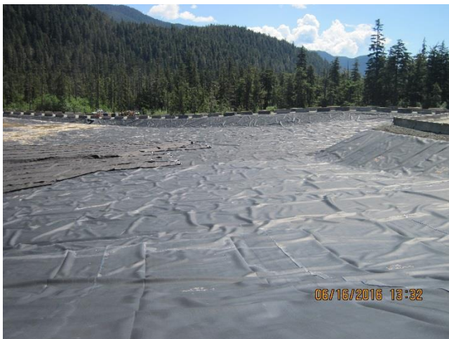
Photo 25. New liner installed for the TDF expansion.
