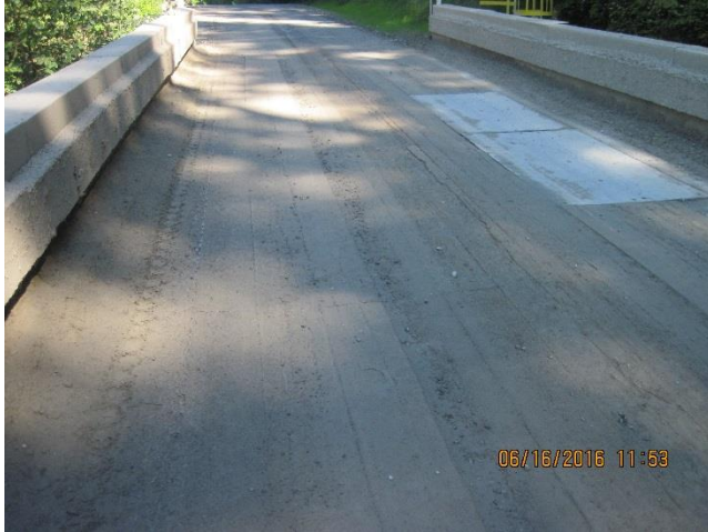
Photo 17. Falls Creek Bridge.
