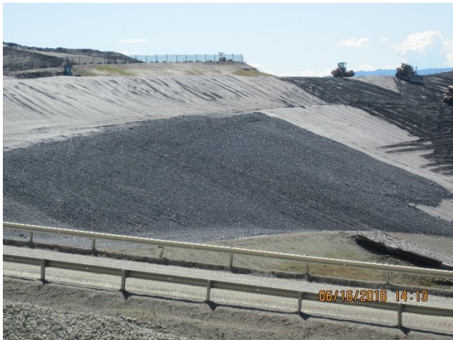
Photo 27. Class 1 rock is placed on the outer slopes at the TDF.
