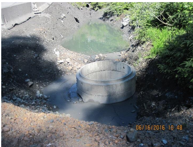
Photo 11. Rock check dam and sump across from BD-01.
