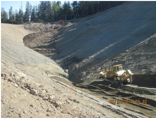
Photo 4. Sand Pit excavation material used for the TDF expansion.
