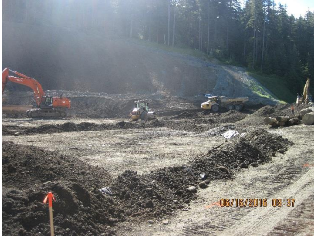
Photo 3. Sand Pit excavation material used for the TDF expansion.
