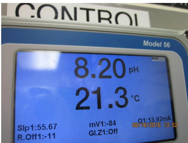
Photo 28. APDES Outfall 002 Control pH.
