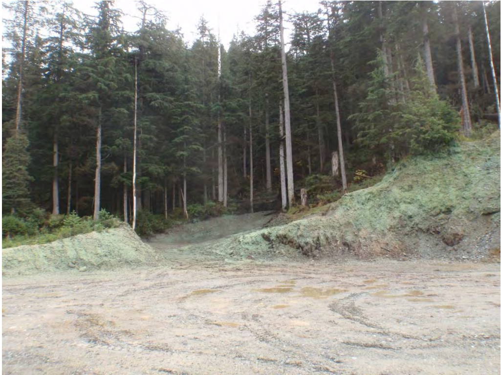
Figure 2.35: 1350 Site - 2013 Production Rock Removal Area
