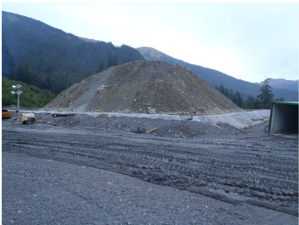
Figure 2.36: Site 23 Temporary Storage Pad for 1350 Material
