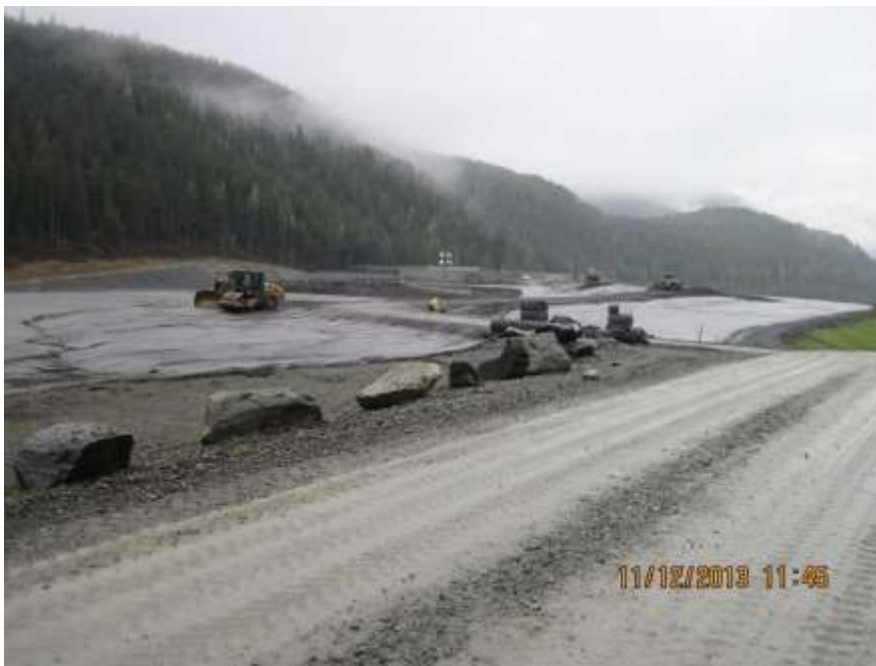
Photo 02. Tailings were being placed in the northwest expansion area on the day of our visit.
