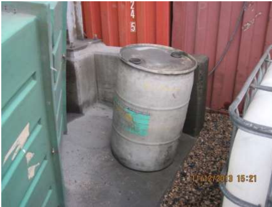
Photo 09. This drum of antifreeze at the powerhouse did not have a lid, and was stored outside of secondary containment.
