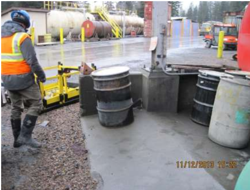
Photo 10. This drum of fuel waste was stored at the powerhouse without secondary containment.
