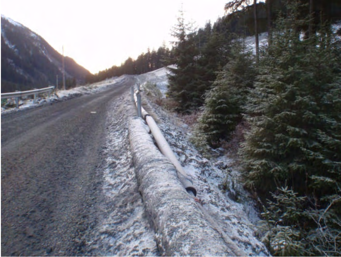
PHOTO 1. Insulation for C Pond Pipeline above B Road, in progress, November 2012
