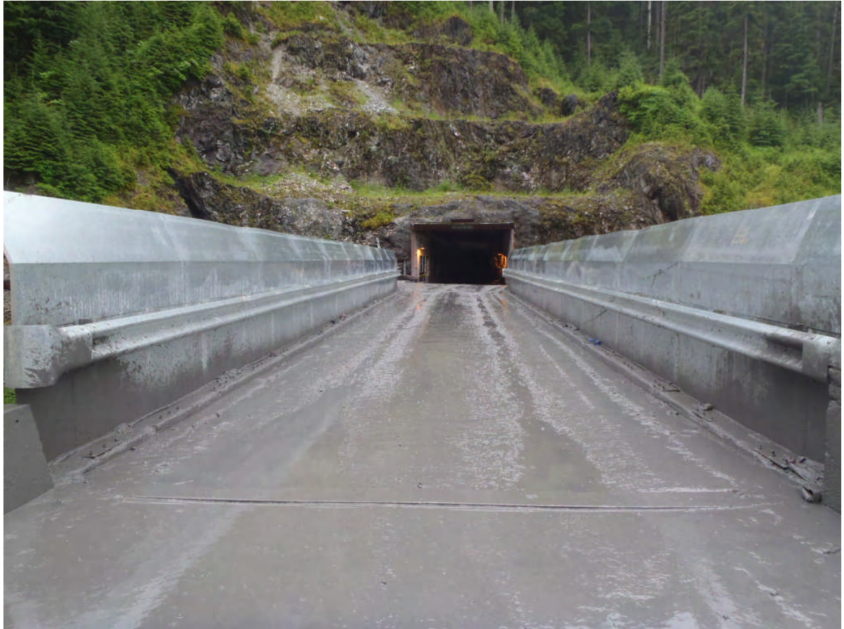
PHOTO 2. New Splash Guards on Greens Creek Bridge, 2012
