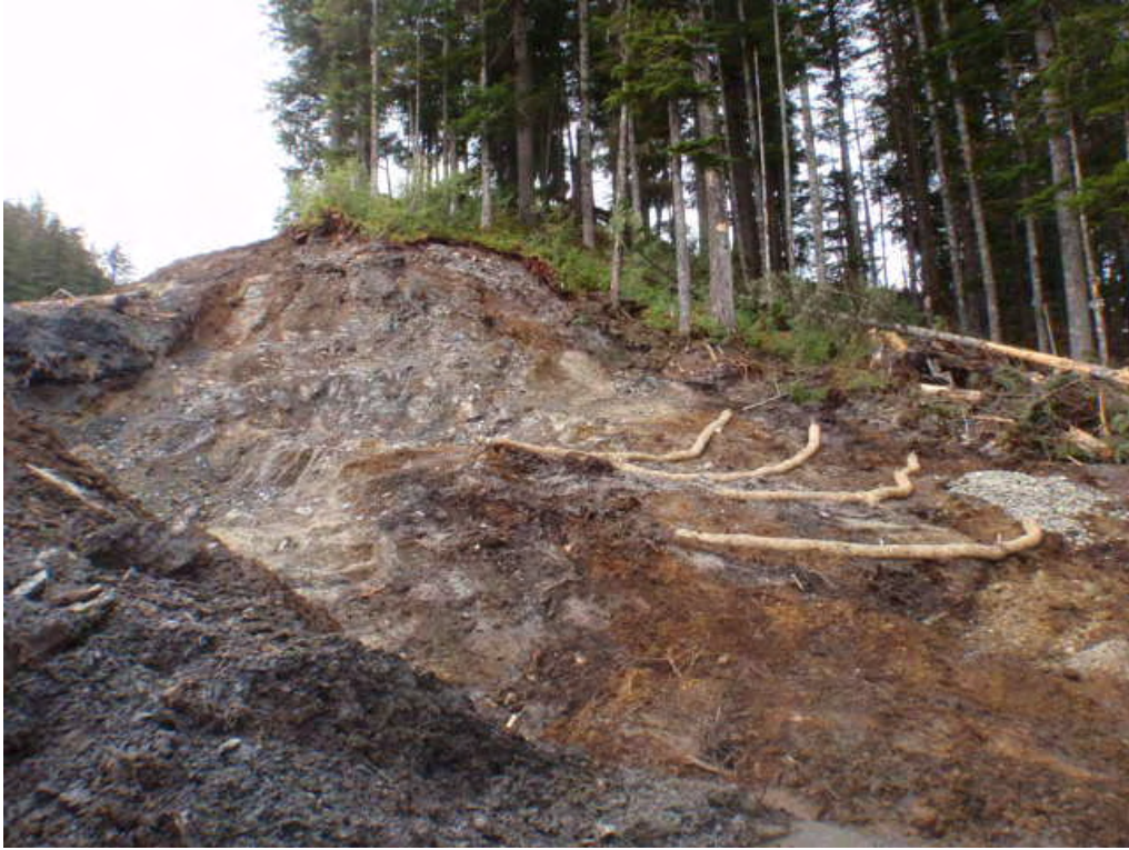
Figure 2.35a 1350 Area - June 2011 During Removal Activities
