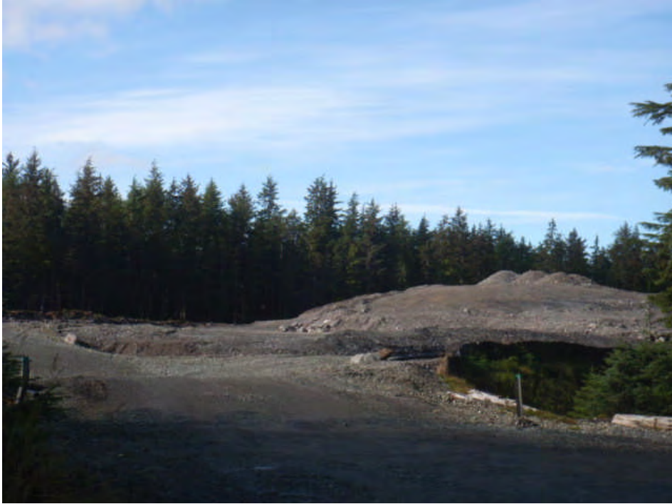
Figure 2.4 Site E Area September 2011
