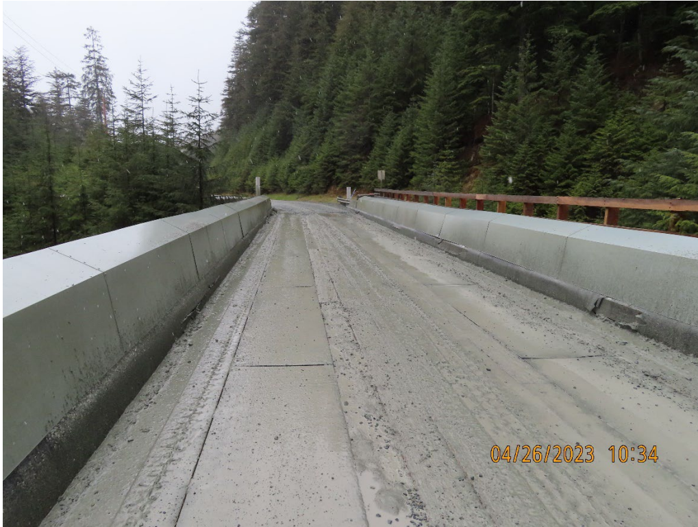
Photo 11. 7.4-mile B Road Bridge (Killer Creek Bridge).
