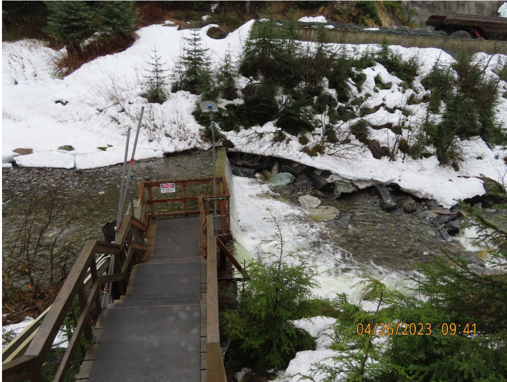
Photo 1). The 920 Greens Creek Weir.
