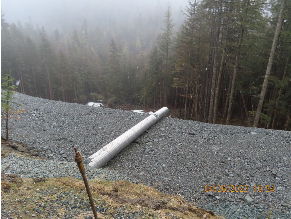
Photo 13. Larger drainpipes were installed during the reconstruction to improve drainage.
