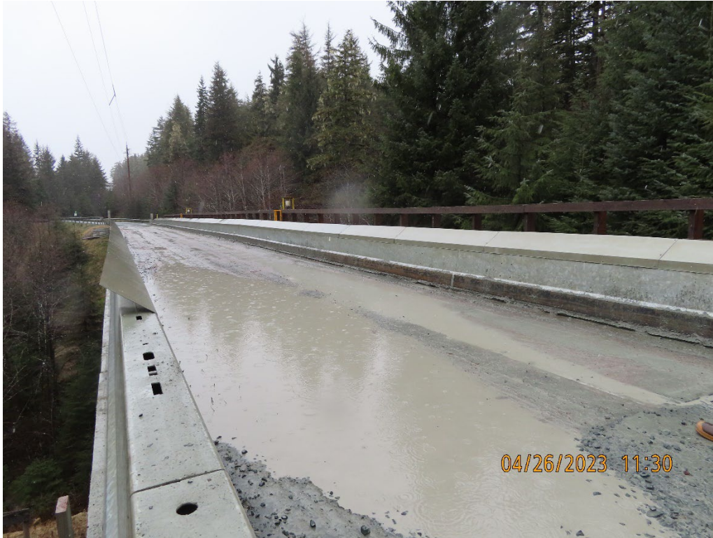
Photo 17. 3.0-mile B Road Bridge (Zinc Creek Bridge).
