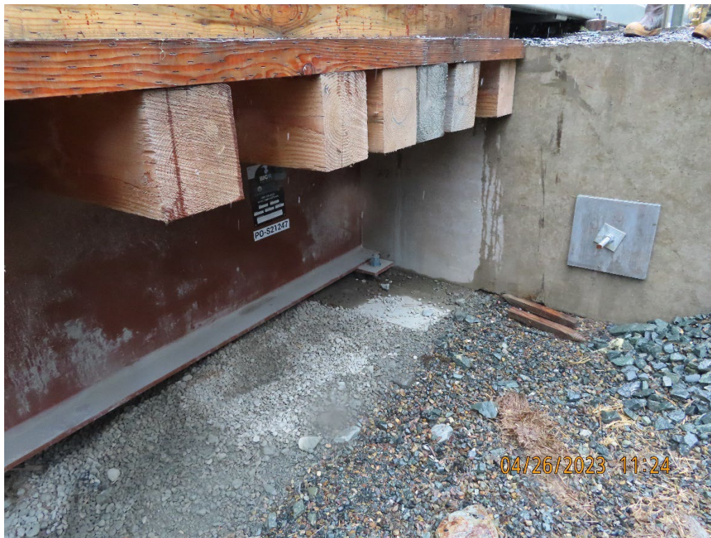
Photo 16. 3.4 B Road Bridge abutment.
