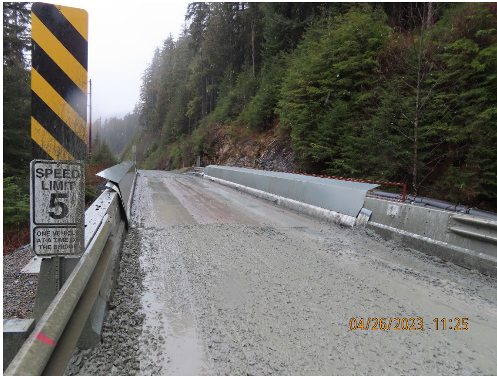
Photo 15. 3.4 B Road Bridge (Falls Creek Bridge).
