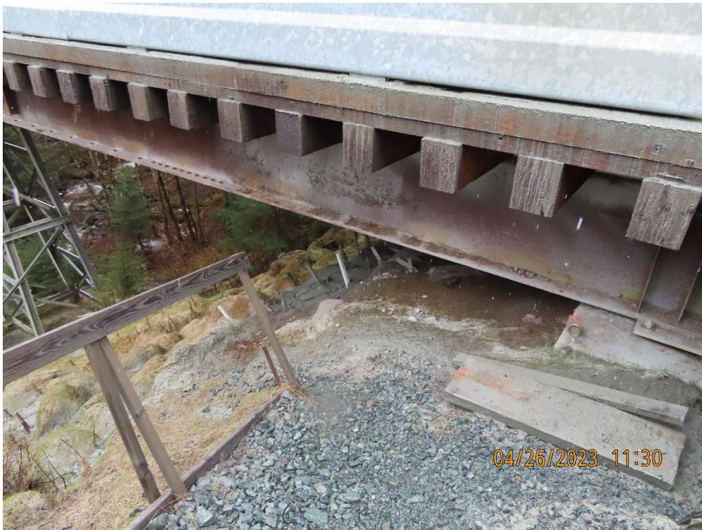
Photo 18. Zinc Creek Bridge abutment.
