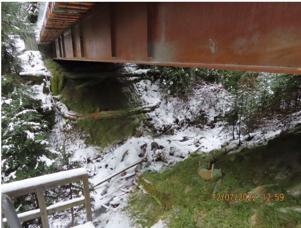
Photo 9. Killer Creek Bridge abutment BMP's.
