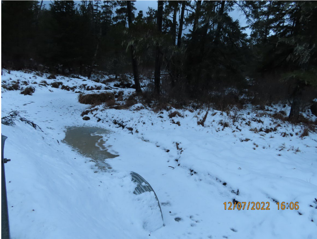
Photo 20. View upstream from new 2.5 mile A-road culvert.
