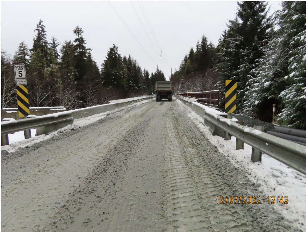
Photo 14. Zinc Creek Bridge.
