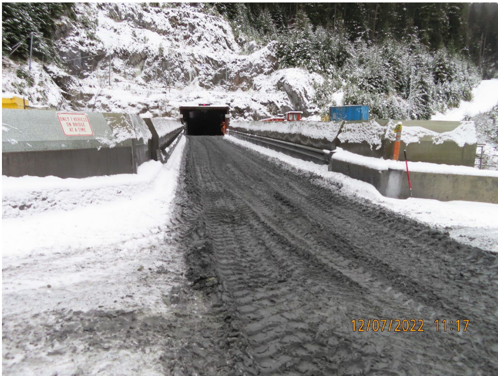
Photo 3. Greens Creek bridge and 920 portal.
