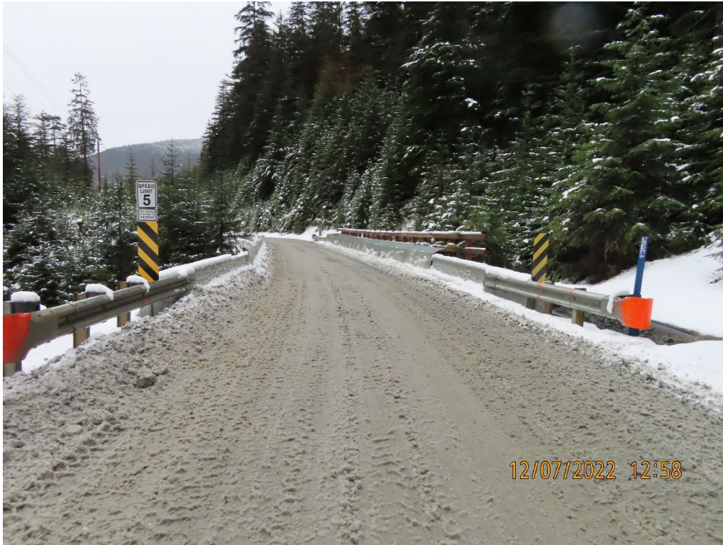
Photo 8. Killer Creek Bridge surface.
