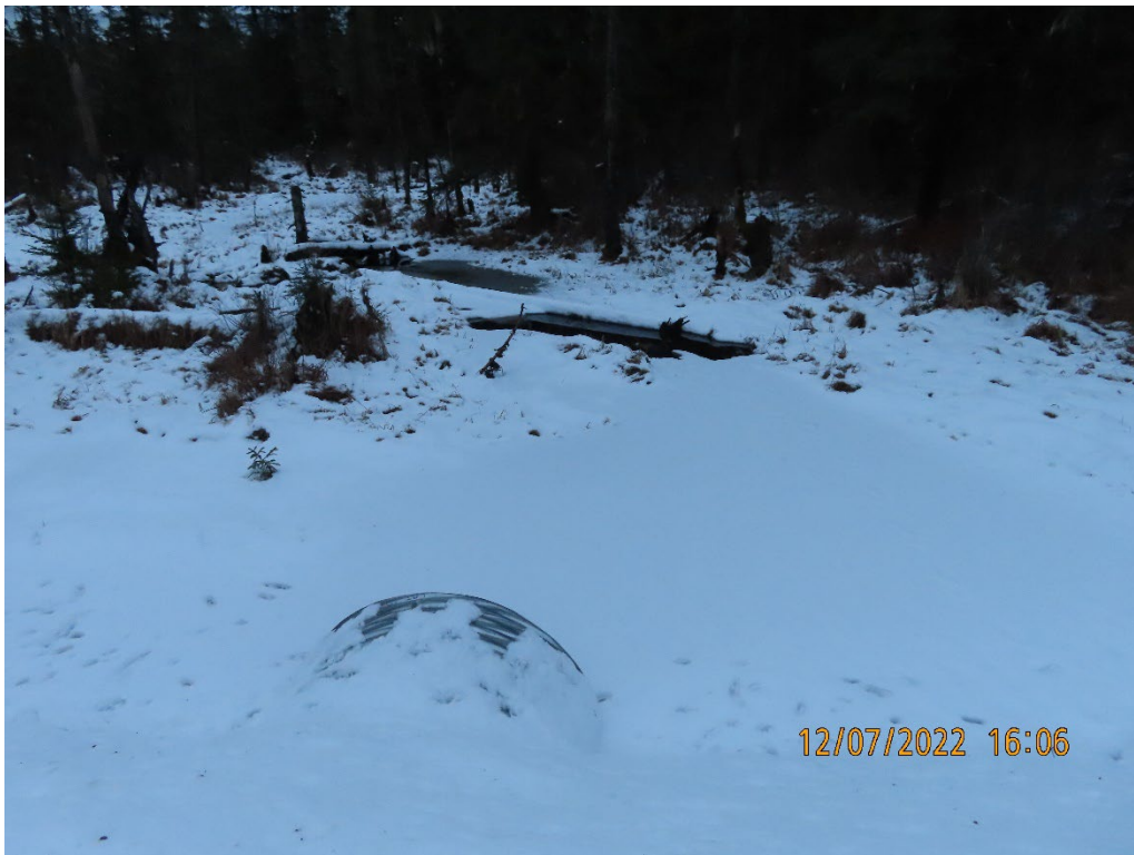
Photo 21. View downstream from new 2.5 mile A-road culvert.
