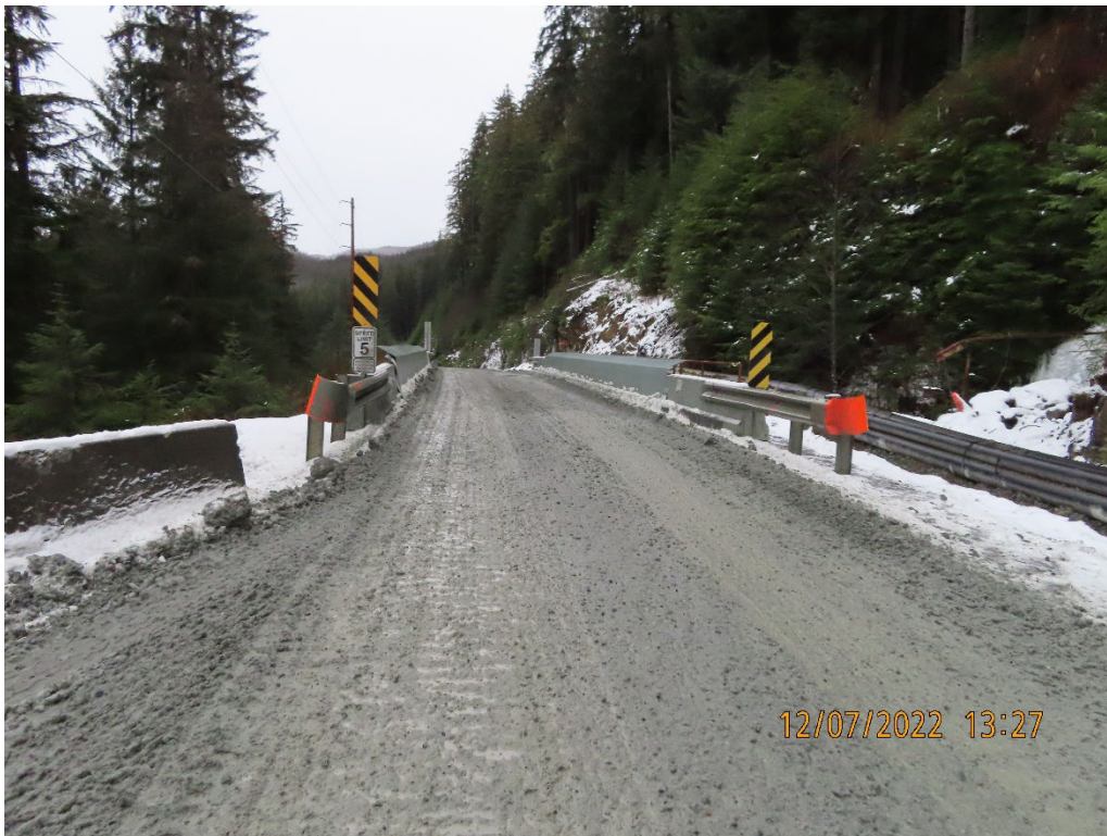
Photo 11. Falls Creek Bridge surface.
