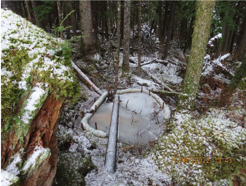
Photo 16. Outlet pipe of the "Gnome Pond" BMPs located adjacent to the Zinc Creek Bridge.
