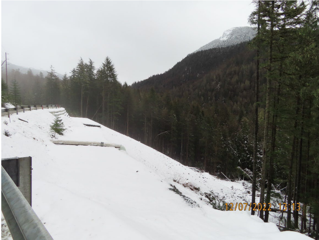
Photo 10. 5.6 mile B-road landslide repairs.
