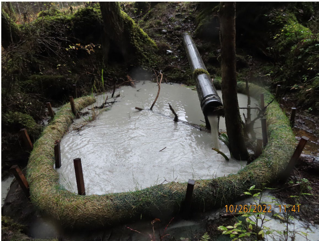
Photo 25. Outlet pipe of the "Gnome Pond" BMPs located adjacent to the Zinc Creek Bridge.
