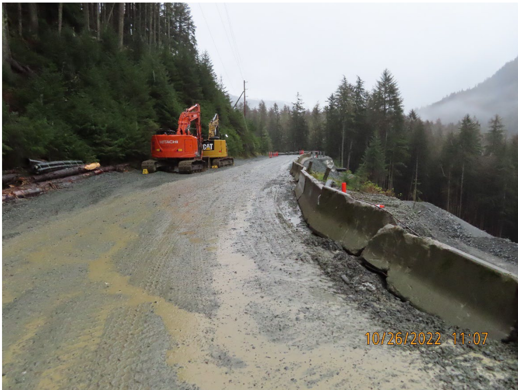
Photo 15. 5.6 mile B-road landslide repairs.
