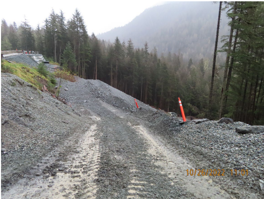
Photo 11. 5.6 mile B-road landslide repairs.
