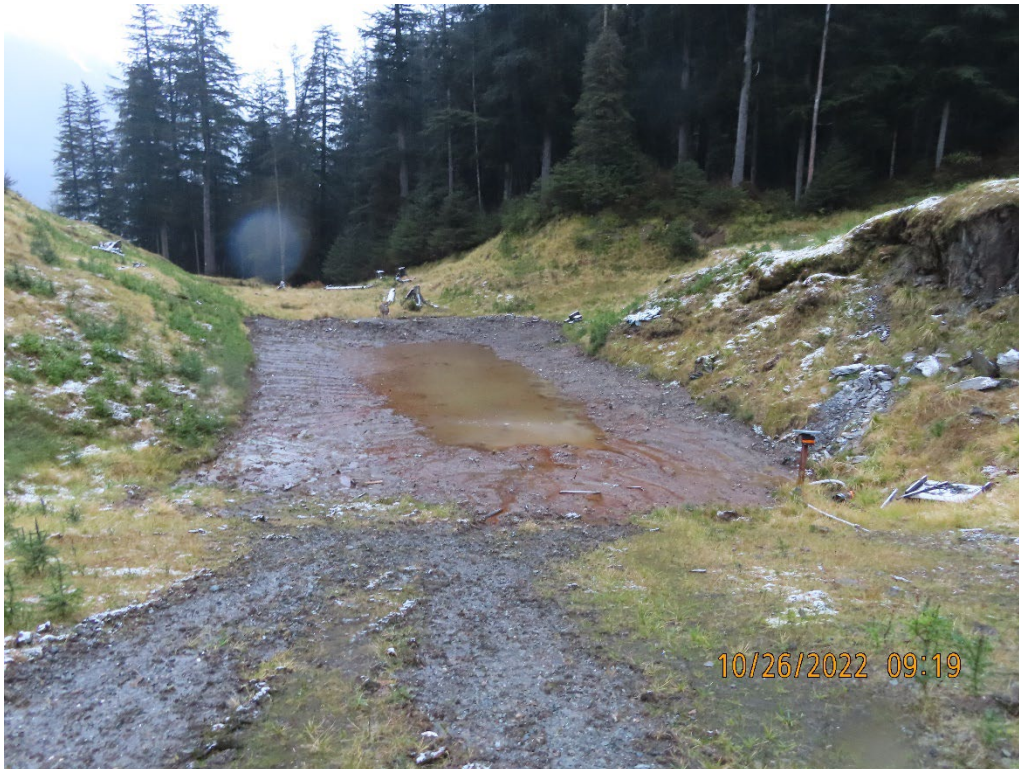
Photo 1. The 1350 area and new water collection sump.
