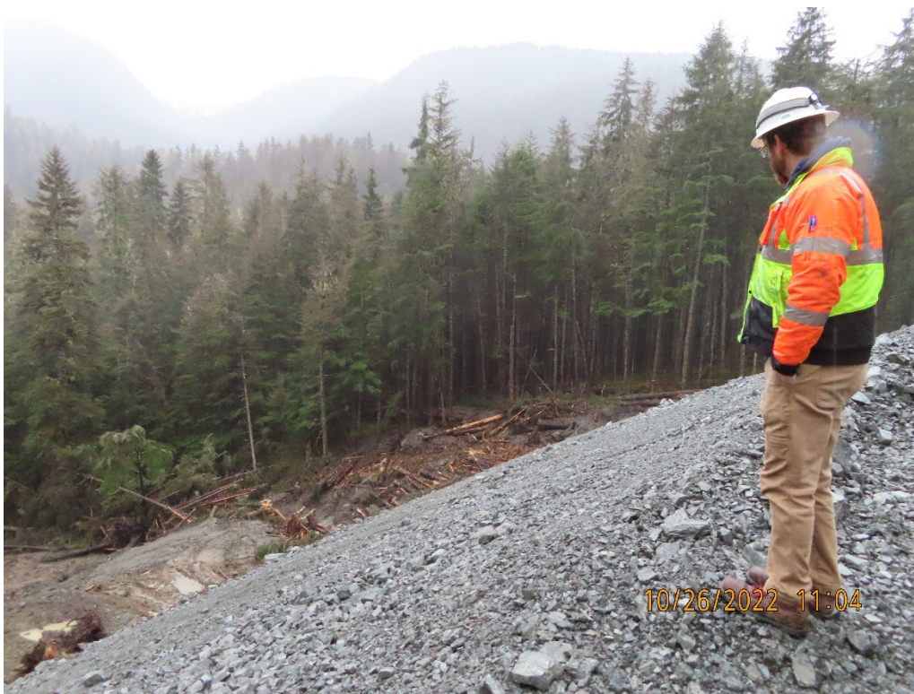
Photo 13. 5.6 mile B-road landslide repairs.
