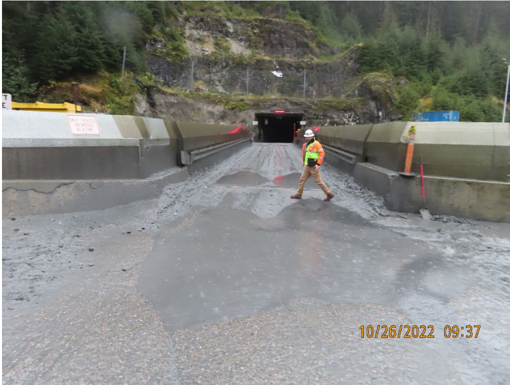
Photo 4. Greens Creek bridge with minor ponding of water.
