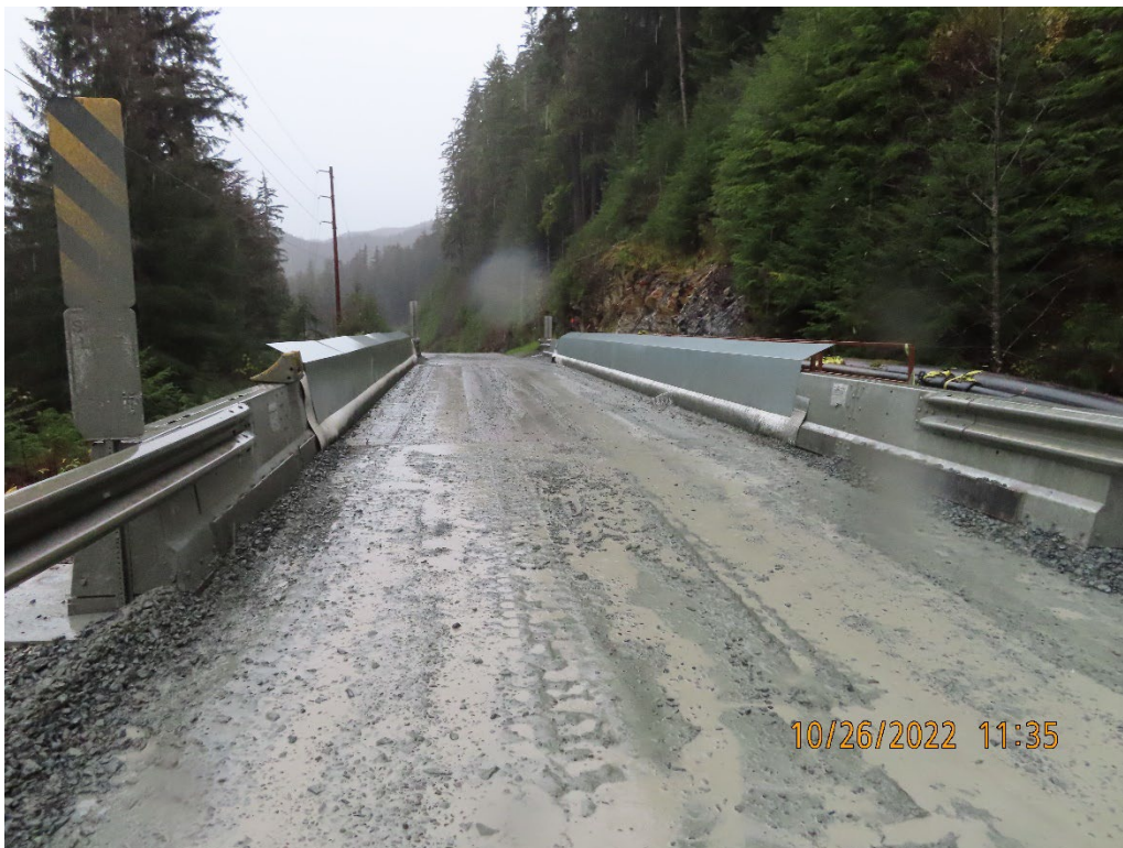
Photo 19. Falls Creek Bridge surface.
