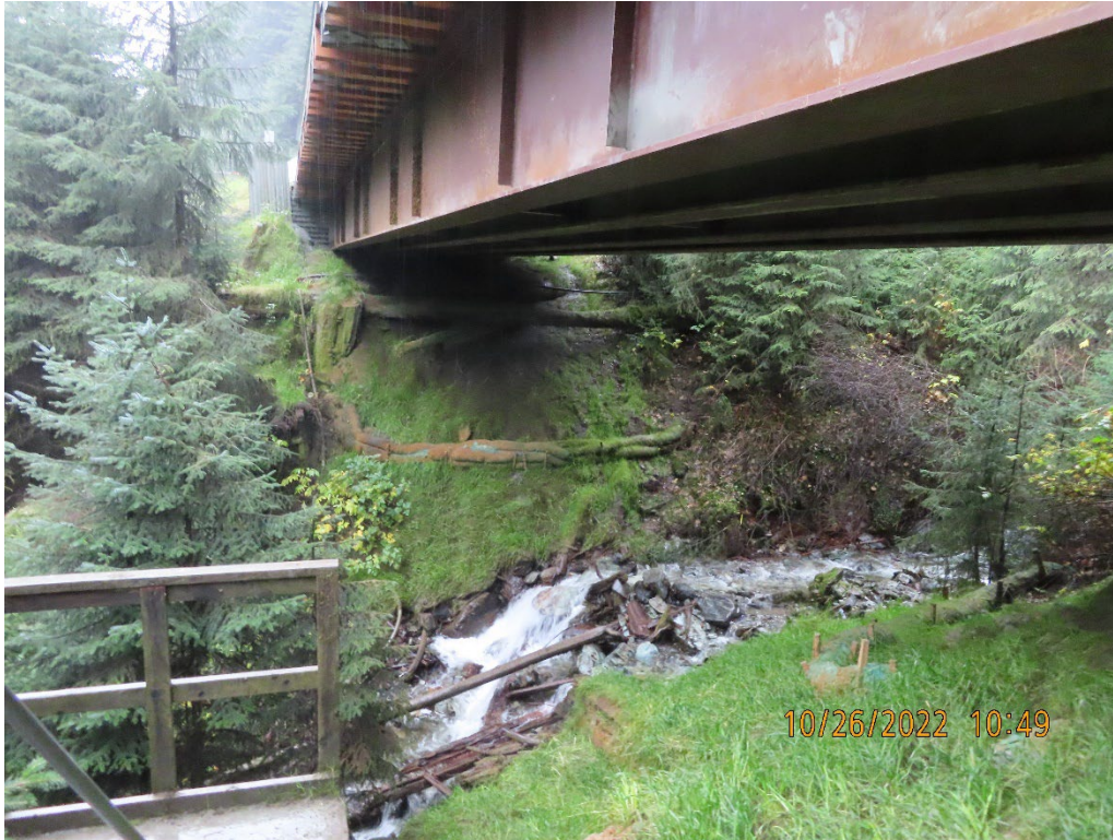
Photo 10. Killer Creek Bridge abutment BMP's.
