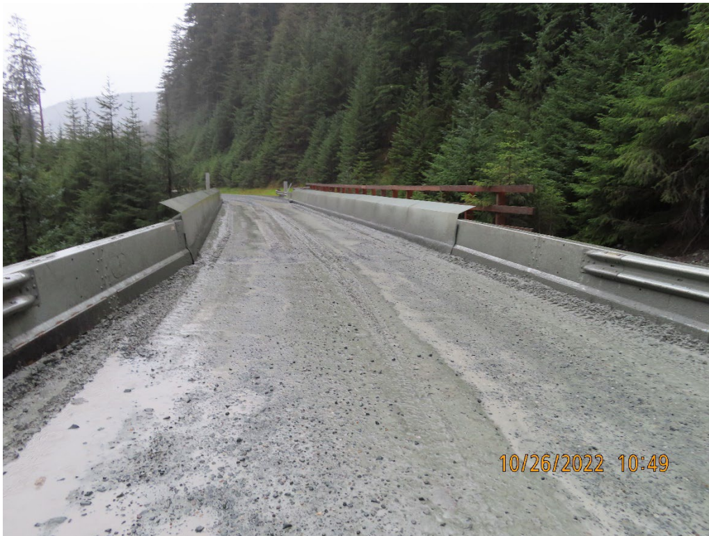
Photo 9. Killer Creek Bridge surface.
