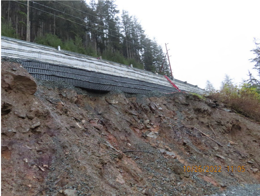
Photo 14. 5.6 mile B-road landslide repairs.
