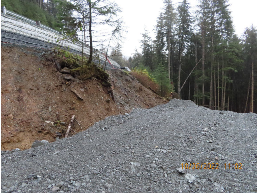
Photo 12. 5.6 mile B-road landslide repairs.
