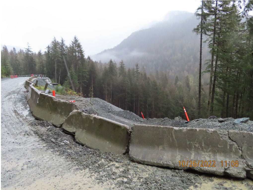
Photo 16. 5.6 mile B-road landslide repairs.
