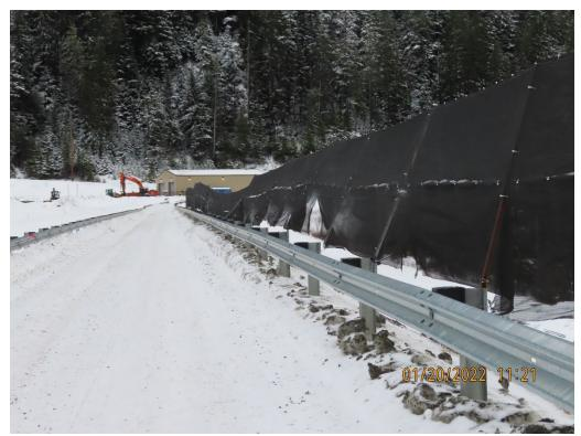
Photo 12. Damaged fugitive dust fencing along southern edge of the TDF.
