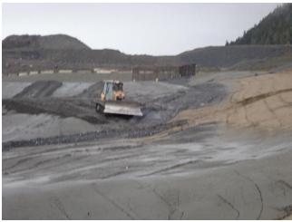
Photo 12. A bulldozer compacting tailings and contouring recently deposited tailings.
