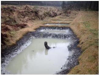
Photo 11. The series of BMPs for stormwater management near the 3.0-mile maker B road.
