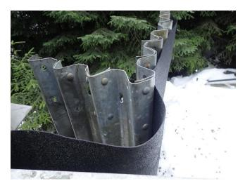
Photo 7. A steel wall was installed along the abutment to prevent erosion.
