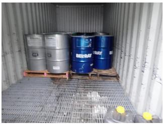
Photo 3. Petroleum products stored with appropriate secondary containment.
