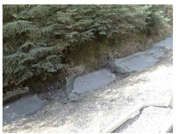
Photo 10. Sediment sump require mucking at the 7.4 mile B-road Bridge.
