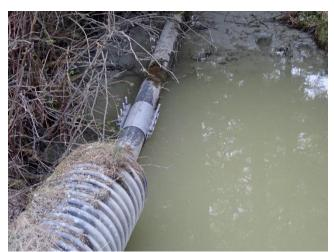
Photo 12. At Site E, a steel clamp was placed over the leaking section of the pipe.
