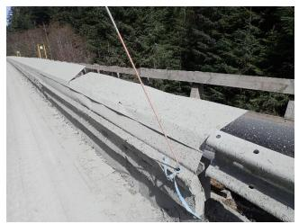
Photo 16. The damaged section splashguard requires repair/replacement.
