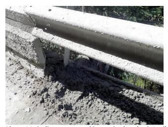
Photo 14. Sediment removal is required at the 3.4 mile B-road bridge ends.
