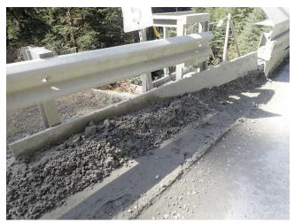
Photo 9. Sediment removal required at Killer Creek Bridge ends.
