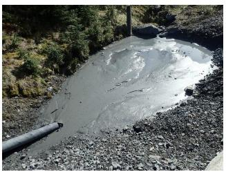
Photo 4. Sediment sump at the base of Ore Pad hill requires mucking.
